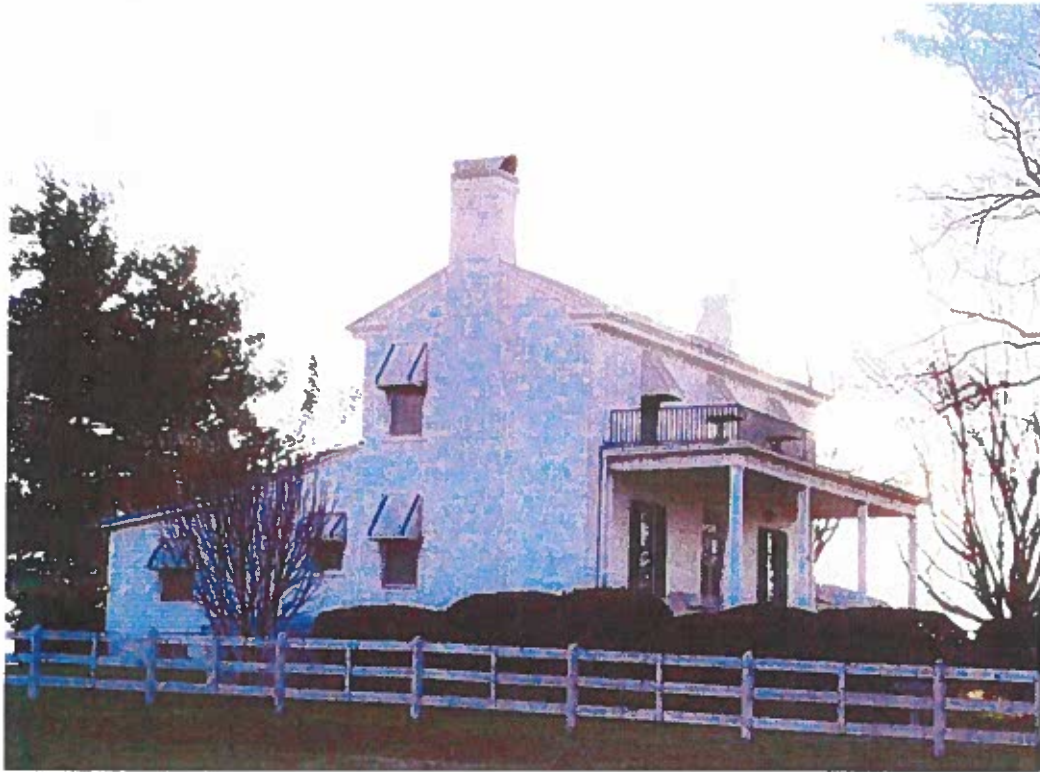
Side view from east
