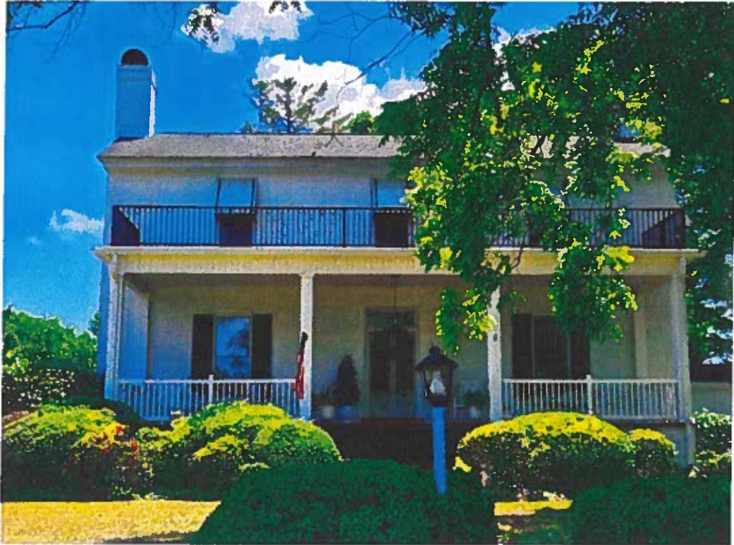
Front view from north
