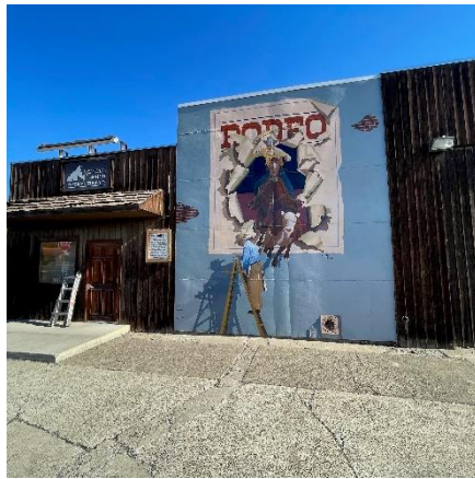
Grade Change West Facade
