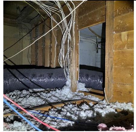
Attic Space Above Southern Portion of Building
