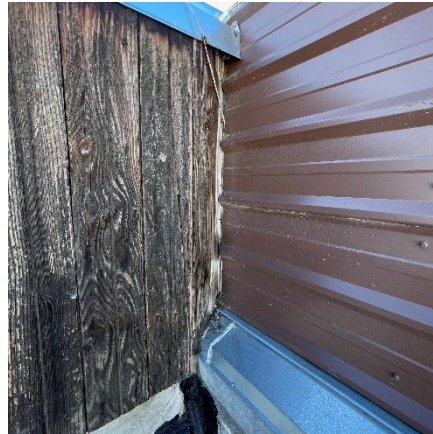
Improper Sealing/Flashing
