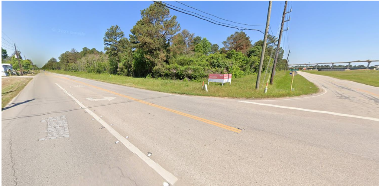
View from Rocky Rd. and Boudreaux Rd.
