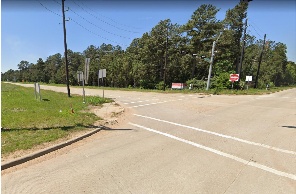
View from Rocky Rd. and SH 99
