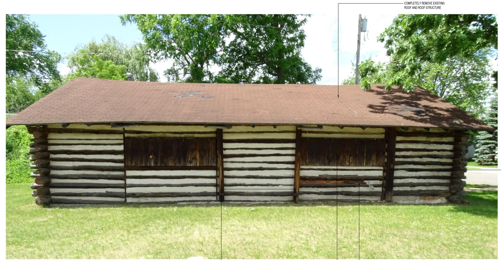
REMOVE EXISTING 4x6 POSTS AFTER ROOF INSTALLATION. PATCH AND MATCH (RESTORE) WALL BEHIND POSTS AS REQUIRED, TYP.
