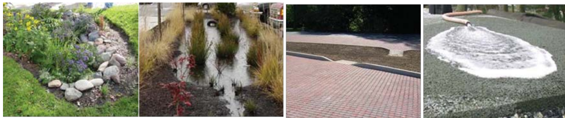
Figure 3.8 demonstrates a few common stormwater management techniques (from left to right): rain garden, bio-swale, pervious pavers, & porous pavement
