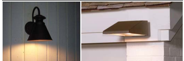
The upper graphic illustrates the different types of lighting techniques from no cutoff to full-cutoff. The lower images provide good examples of full-cutoff building light fixtures.
