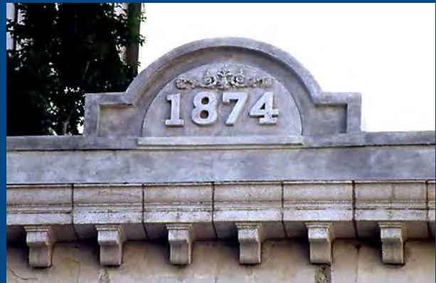
APPROPRIATE An example of a reconstructed architectural pediment.
