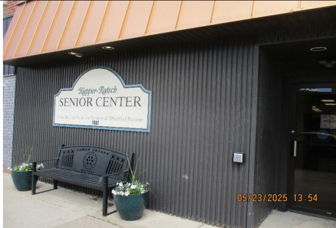
Front entry on Superior Avenue
