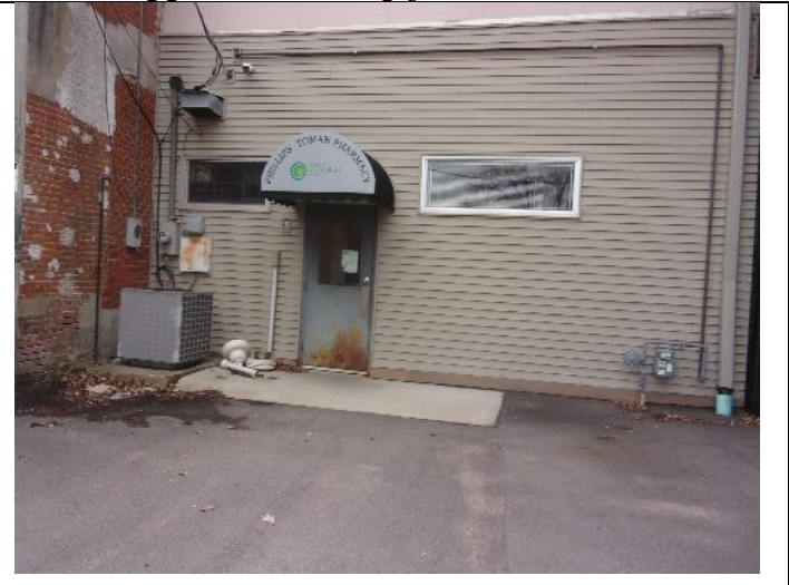
Back of building 1004 Superior Ave.
