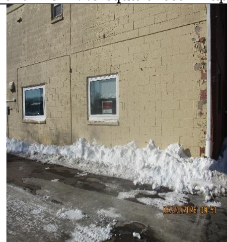
Alley side of building 107 Milwaukee Street
