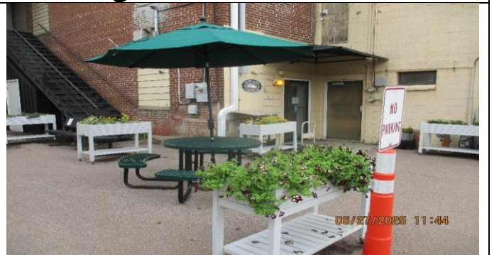
Back (main) entry across alley from WWTC parking lot.
