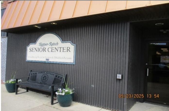
Front entry on Superior Avenue
