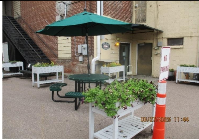
Back (main) entry across alley from WWTC parking lot.
