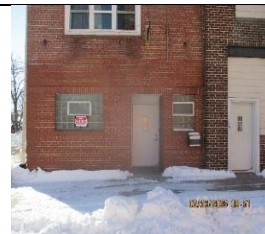
Front of building 107 Milwaukee Street
