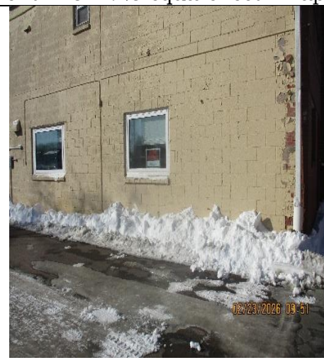
Alley side of building 107 Milwaukee Street
