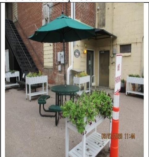
Back door side of building 107 Milwaukee Street
