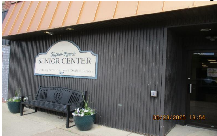
Front entry on Superior Avenue
