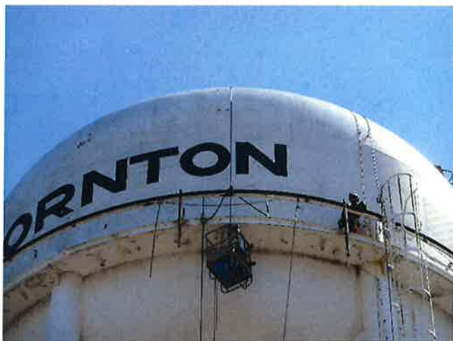
CATWALK RAIL EXTENSION IN PROCESS
