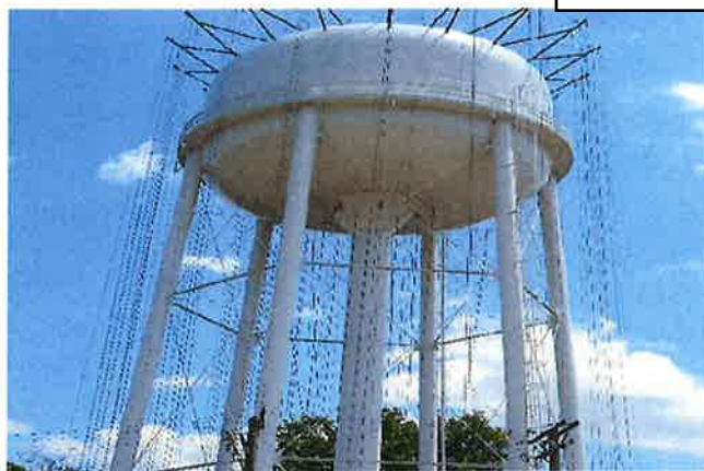
INTERMEDIATE COAT COMPLETED
