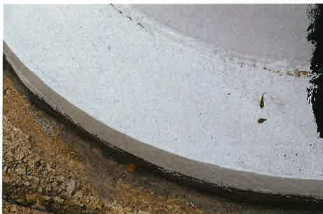
CONCRETE AREAS AROUND BASES HAVE BEEN REPAIRED/COATED
