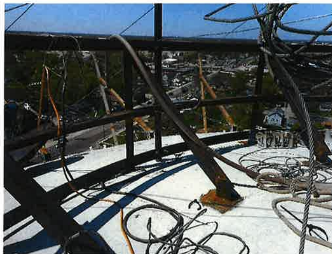
ROOF CORRAL FABRICATION COMPLETED
