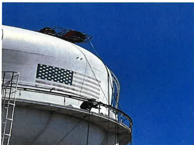
CATWALK RAIL EXTENSION IN PROCESS
