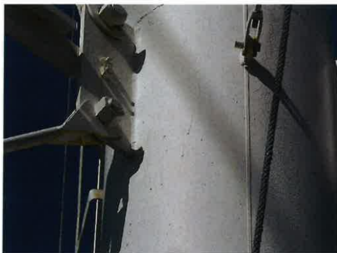
RUNS IN COATING PREVIOUS APPLICATION
