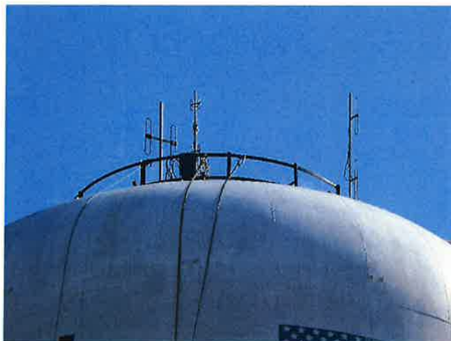
NEW ROOF CORRAL INSTALLATION
