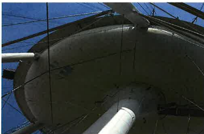
SPOT SANDBLASTED AREAS OF CORROSION ON TANK EXTERIOR
