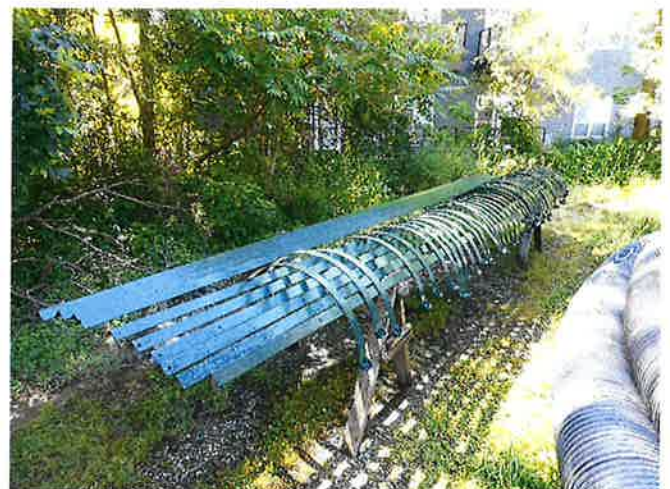
ANGLE IRON CLEANED AND COATED
