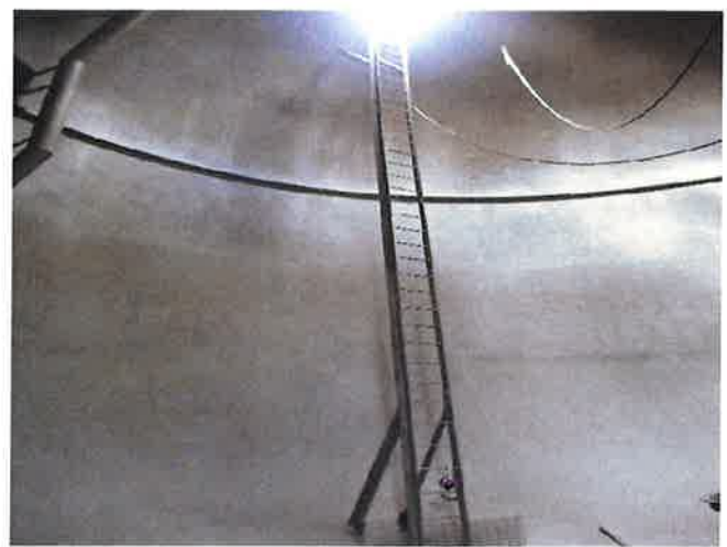
PRIMER COATING IN PROCESS
