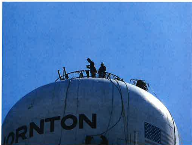
ROOF CORRAL FABRICATION IN PROCESS
