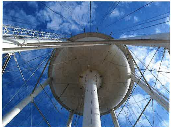
TANK EXTERIOR WATERJET CLEANED
