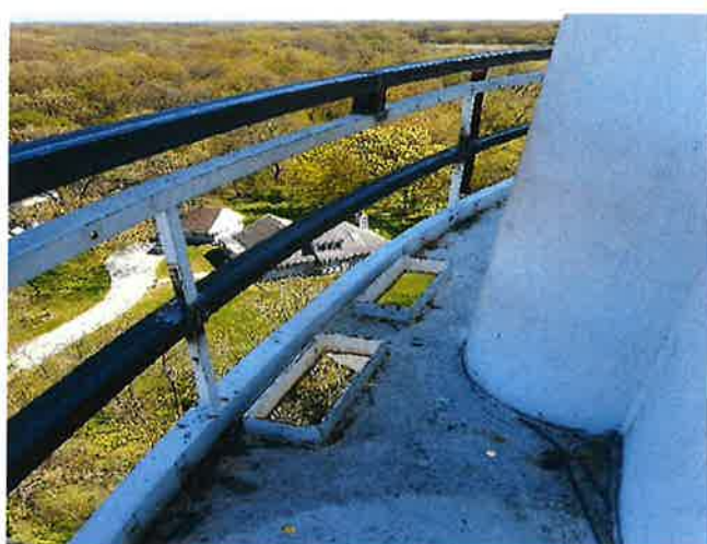
CATWALK HANDRAIL RAISED TO 42"
