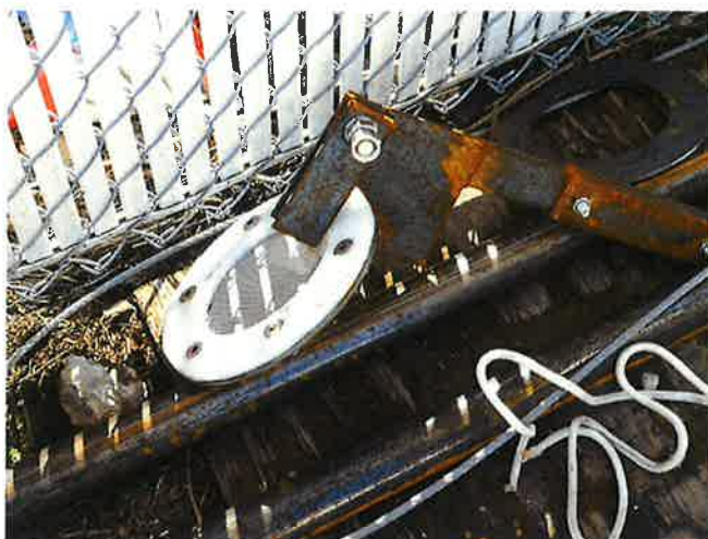
NEW OVERFLOW FLAP GATE
