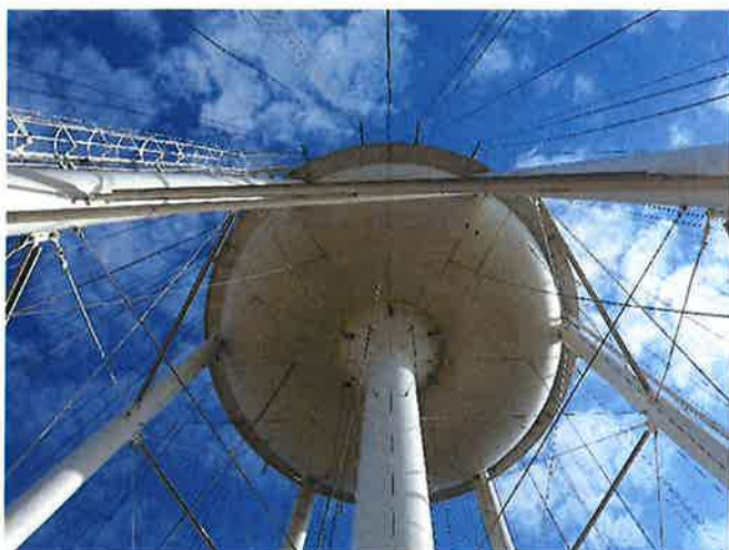
TANK POWER WASHED
