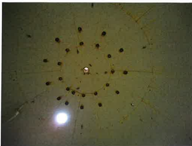
OLD CP PORTS TO BE COVERED WITH WELDED PLATES
