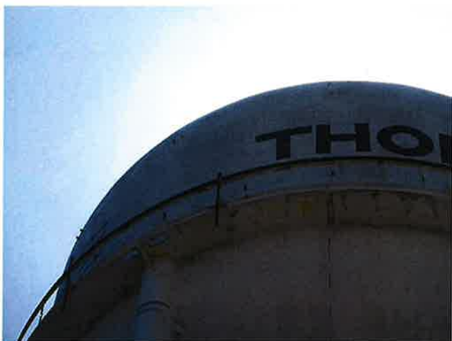
CATWALK RAIL EXTENSION IN PROCESS
