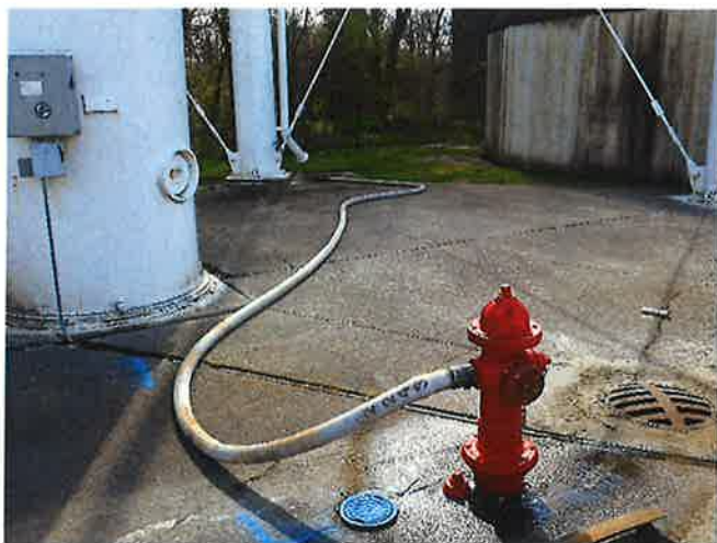
DRAINING OF TOWER IN PROGRESS
