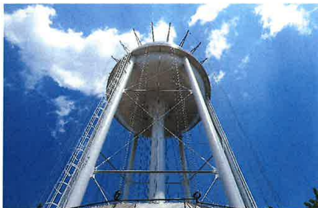
INTERMEDIATE COAT COMPLETED
