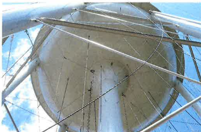
INTERMEDIATE COAT COMPLETED
