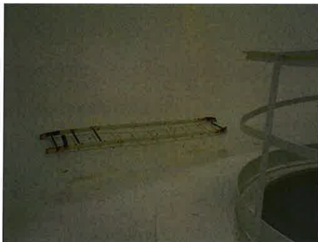
WET INTERIOR LADDER CORRODED AND DETACHED FROM WALL
