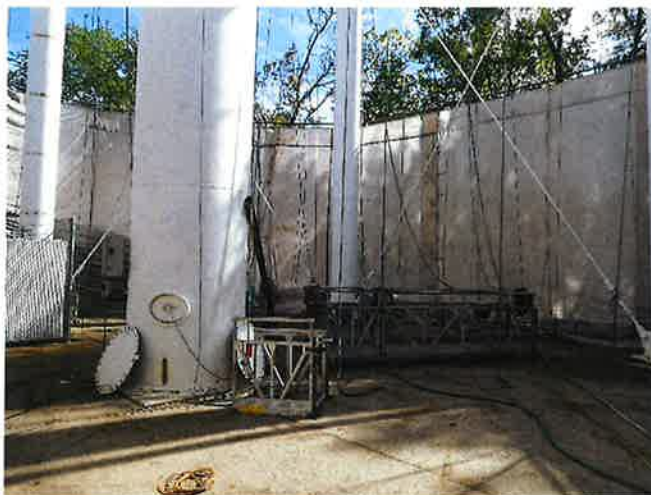
TANK EXTERIOR WATERJET CLEANED
