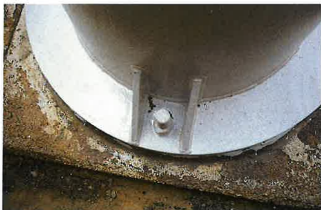
ANCHOR BOLTS AFTER SANDBLASTING
