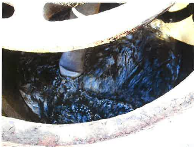
DRAINING OF TOWER IN PROGRESS
