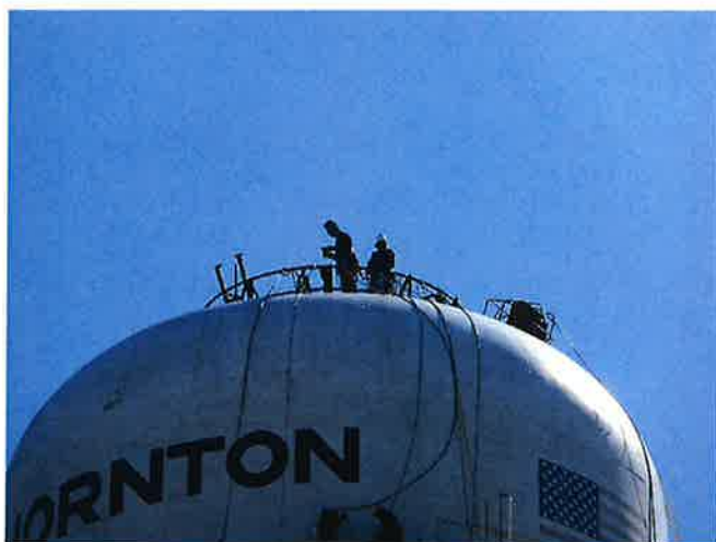
ROOF CORRAL FABRICATION IN PROCESS
