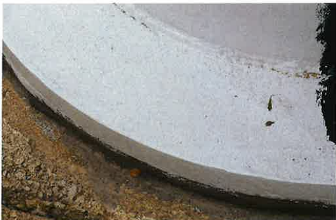
CONCRETE AREAS AROUND BASES HAVE BEEN REPAIRED/COATED
