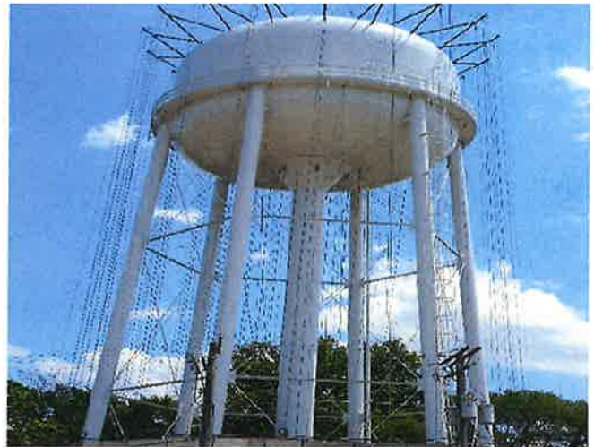
INTERMEDIATE COATING IN PROCESS
