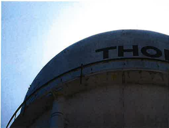
CATWALK RAIL EXTENSION IN PROCESS
