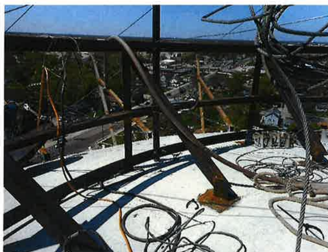
ROOF CORRAL FABRICATION COMPLETED
