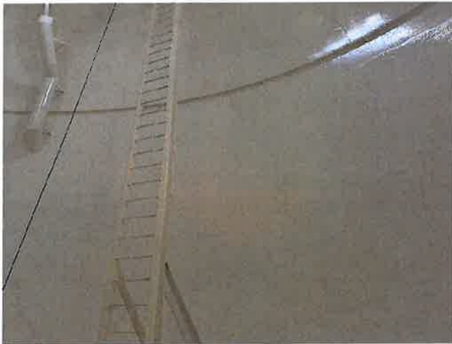
COMPLETED TOPCOAT APPLICATION
