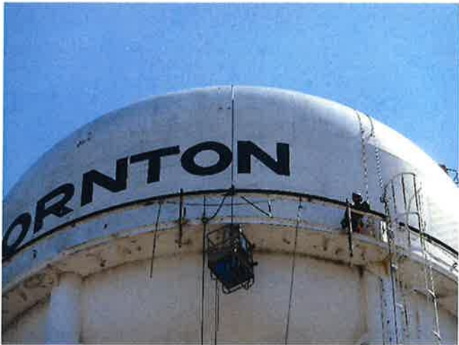
CATWALK RAIL EXTENSION IN PROCESS
