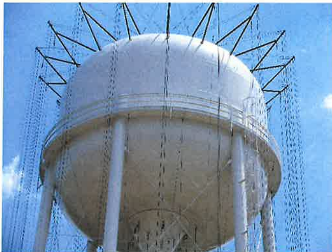
INTERMEDIATE COATING IN PROCESS
