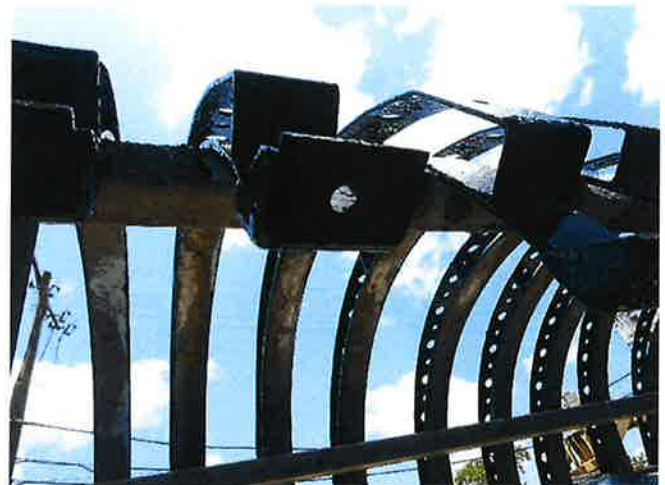
METAL BANDS CLEANED AND COATED
