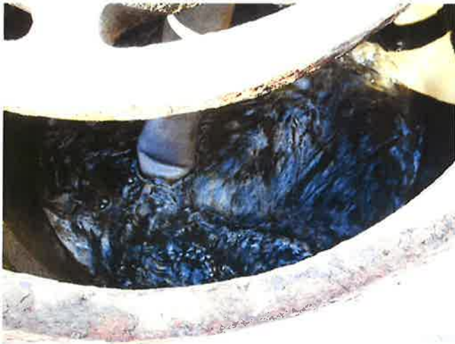
DRAINING OF TOWER IN PROGRESS
