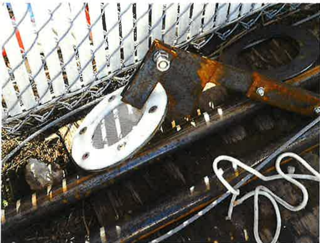
NEW OVERFLOW FLAP GATE
