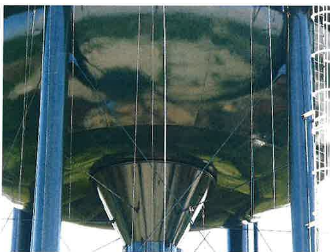
FLOUROPOLYMER TOPCOAT IN PROCESS
