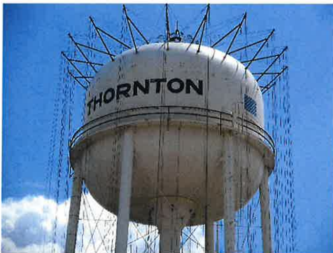
CONTAINMENT SYSTEM INSTALLED
