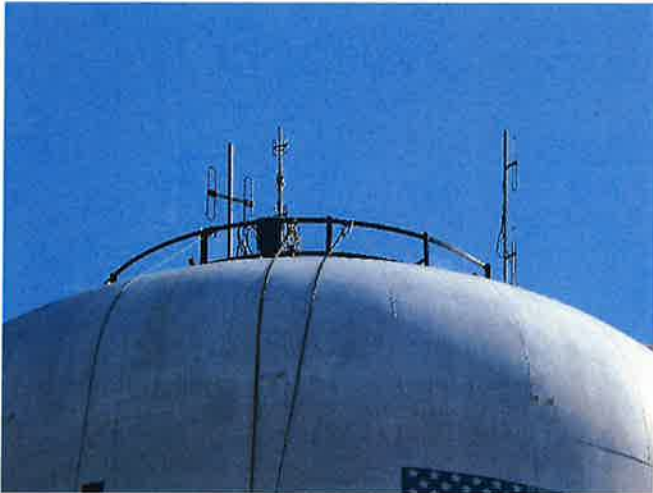
NEW ROOF CORRAL INSTALLATION
