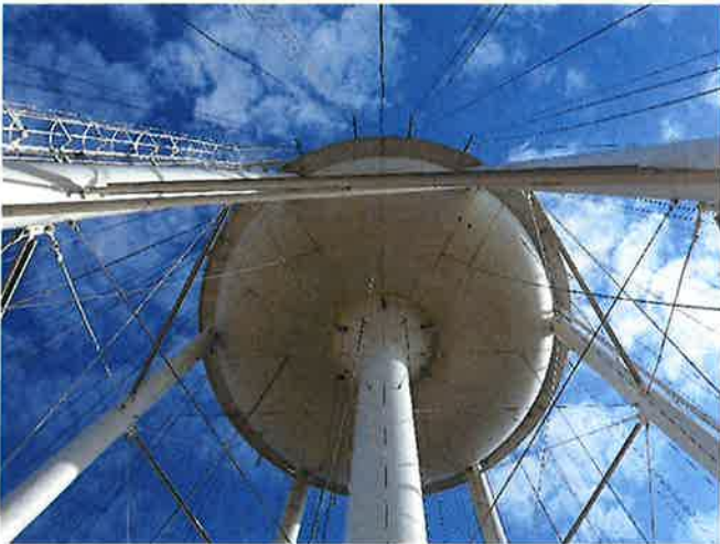
TANK POWER WASHED
