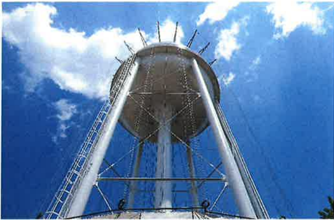
INTERMEDIATE COAT COMPLETED
