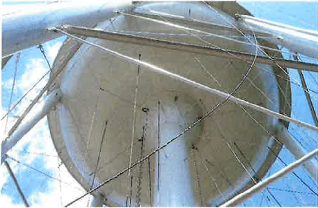
INTERMEDIATE COAT COMPLETED
