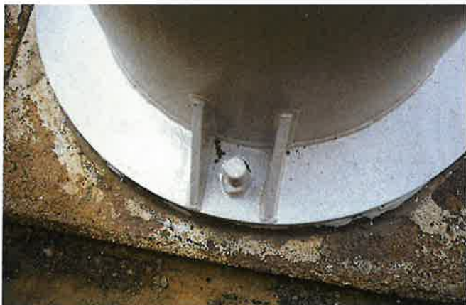
ANCHOR BOLTS AFTER SANDBLASTING
