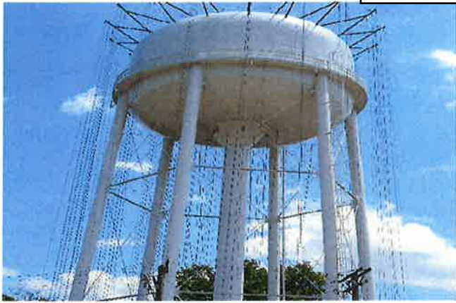
INTERMEDIATE COAT COMPLETED
