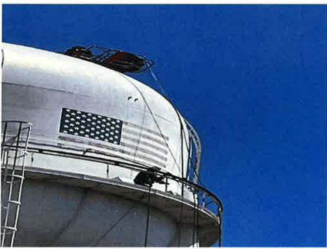
CATWALK RAIL EXTENSION IN PROCESS
