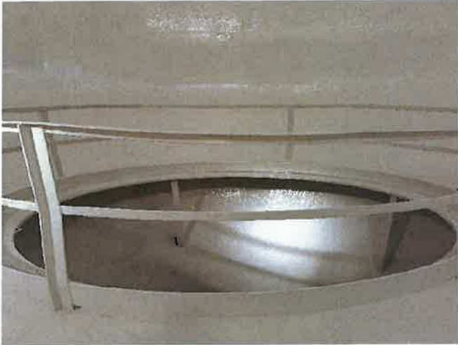
TOPCOAT IN PROCESS
