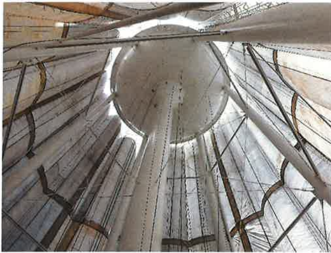
INTERMEDIATE COATING IN PROCESS
