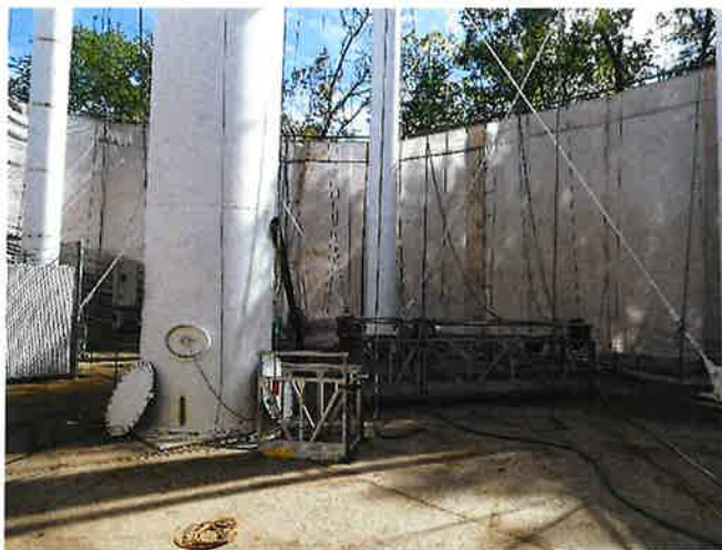
TANK EXTERIOR WATERJET CLEANED
