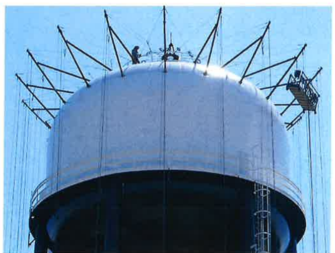
FLOUROPOLYMER TOPCOAT IN PROCESS
