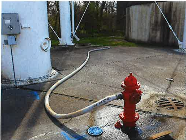
DRAINING OF TOWER IN PROGRESS
