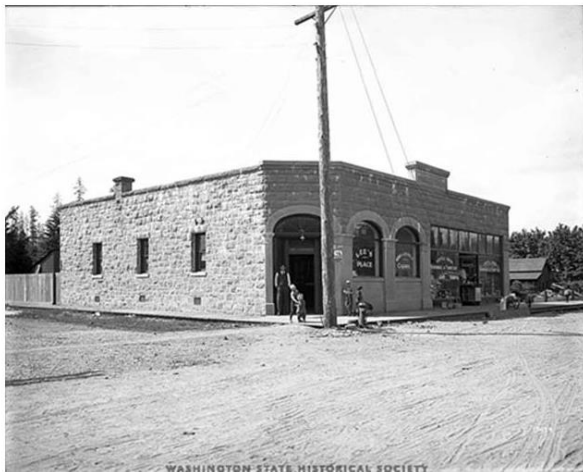
Larger historic structures, like the Columbia Building, were articulated into distinct segments, rather than appearing as one large building. In the Columbia Building, this articulation was accomplished through the creation of two distinct storefronts distinguished by drastically different window arrangements.
