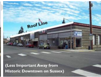
Similar Roof Lines
