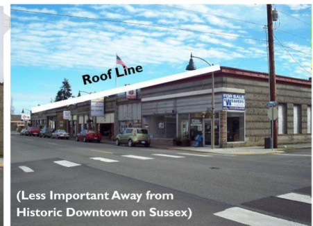
Similar Roof Lines
