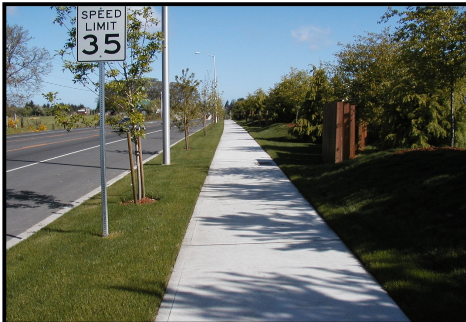
Photo E. View of a well-designed planter strip, however tree wells are not adequate – turf is too close to tree's rootball.
