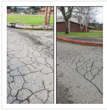
Parking Lot Repairs
