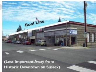
Similar Roof Lines
