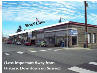
Similar Roof Lines
