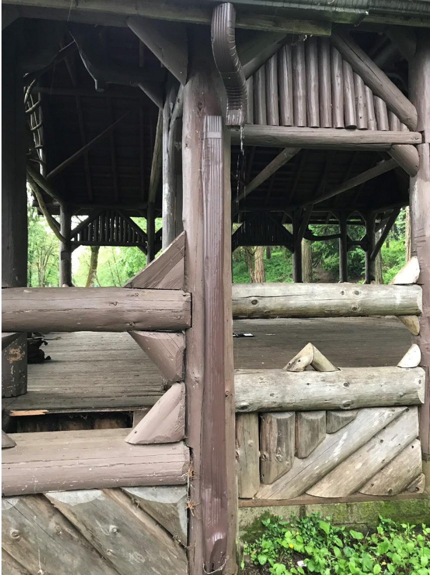
Picture 11 – damaged downspout
