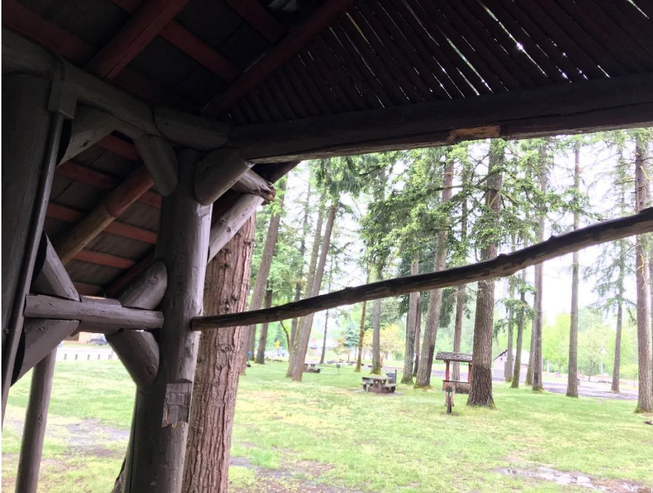
Picture 12 – knee brace removed
