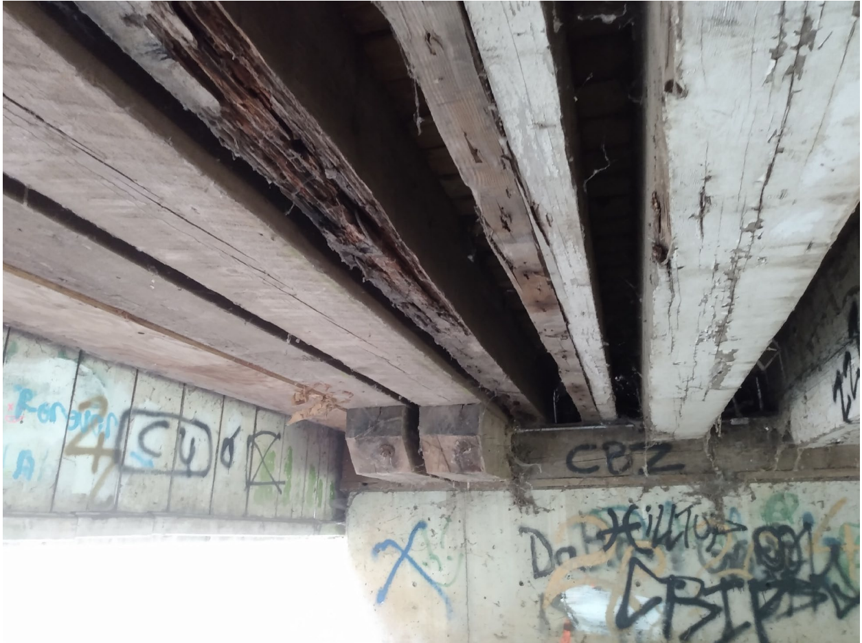
Figure 10 - Bottom chord and stringer 1, 2 and 3
