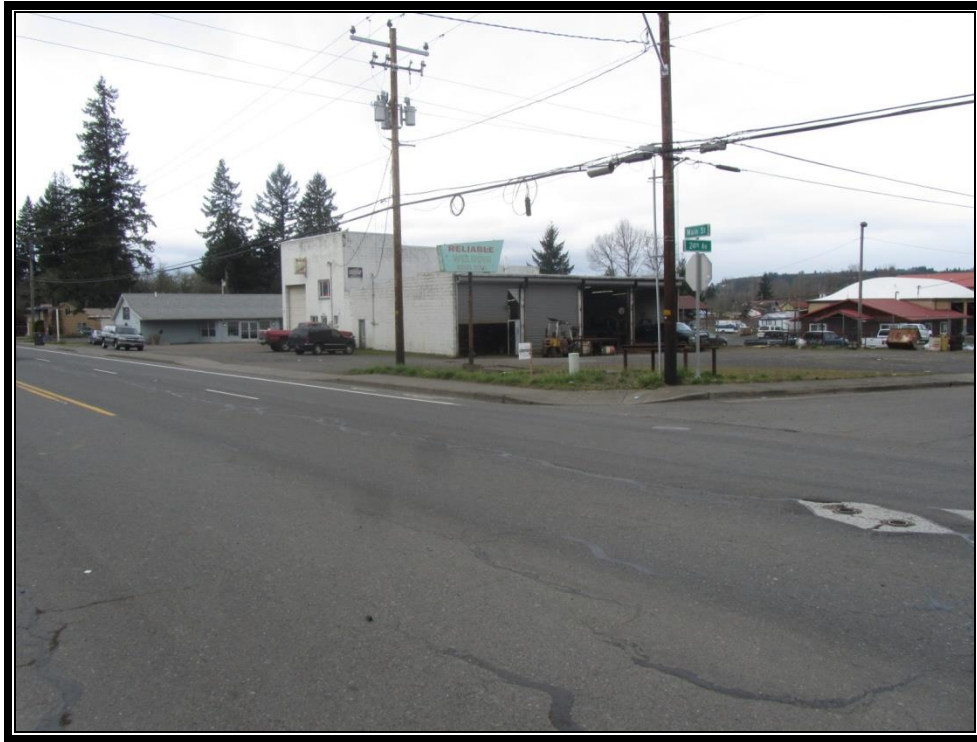
View of Hutchins Trust/Reliable Welding Property taken from 24 th Avenue & Main Street intersection. (A12-491)
