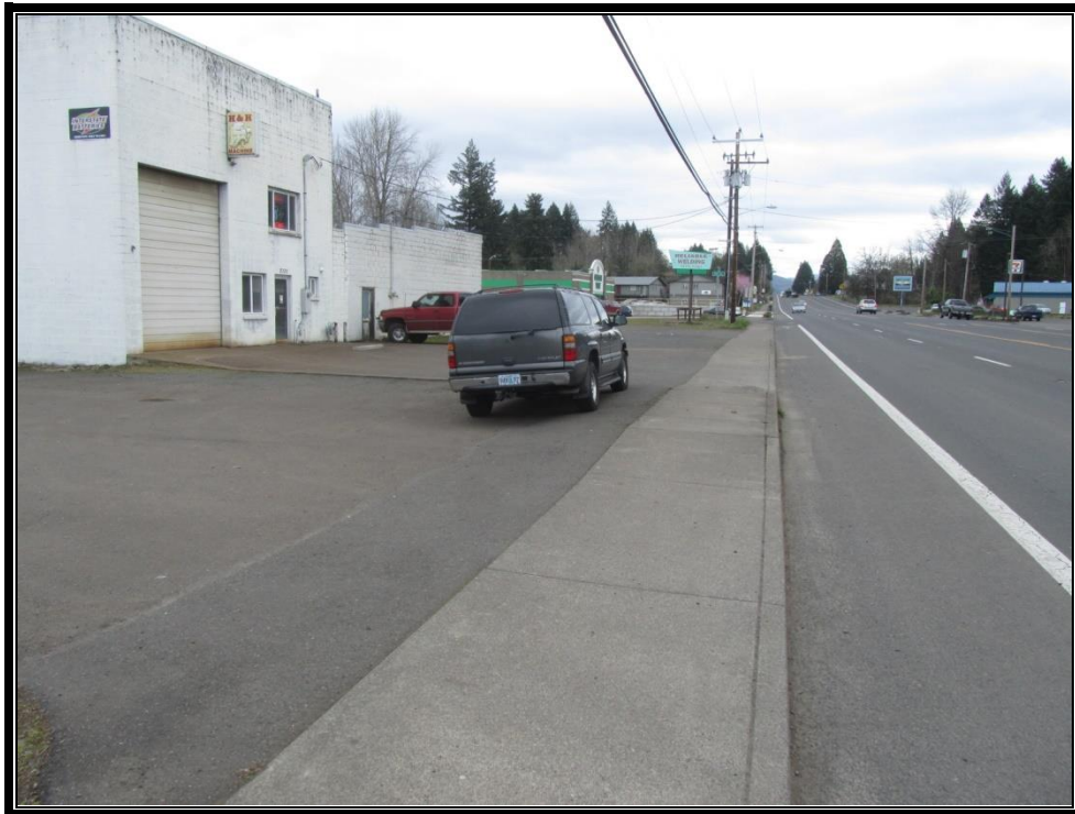
Easterly view of property's Main Street frontage. (A12-487)
