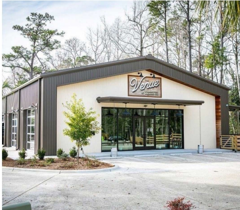
A brewery or food-related manufacturer could locate their facility within employment industrial employment areas.
