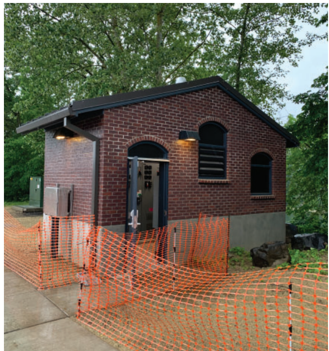
West Yost’s design for the City of Albany’s Riverfront Interceptor Lift Station successfully addresses significant operational and regulatory risks from sanitary sewer overflows (SSOs).
