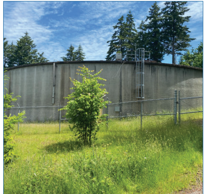
An early project to be evaluated by the City Engineer is the location of a new water storage tank to help address ongoing pressure issues in several areas of the City.
