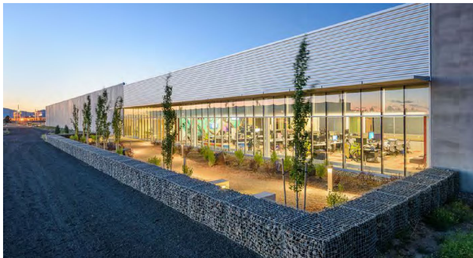
The newest Meta data center in Prineville is LEED Gold certified.
