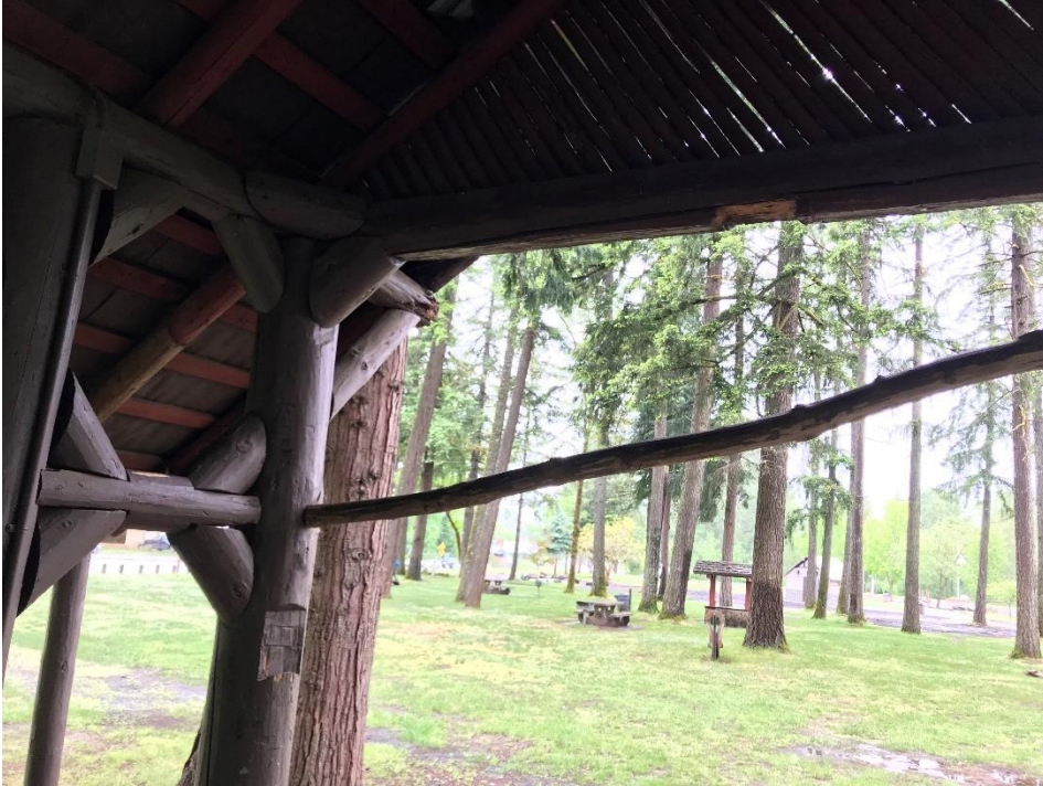
Picture 12 – knee brace removed
