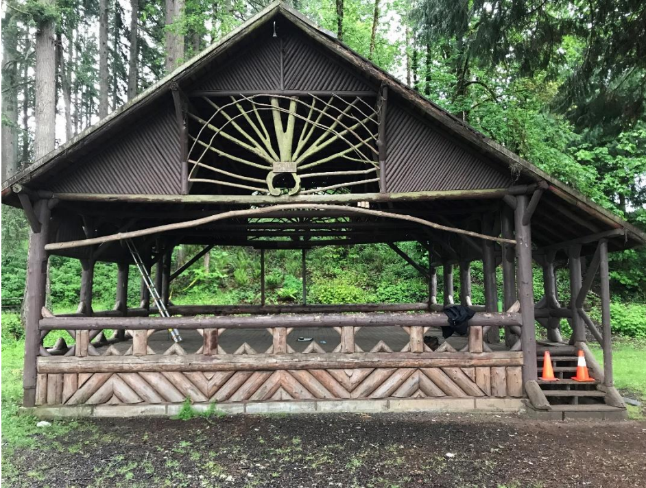
Picture 1 – north side
