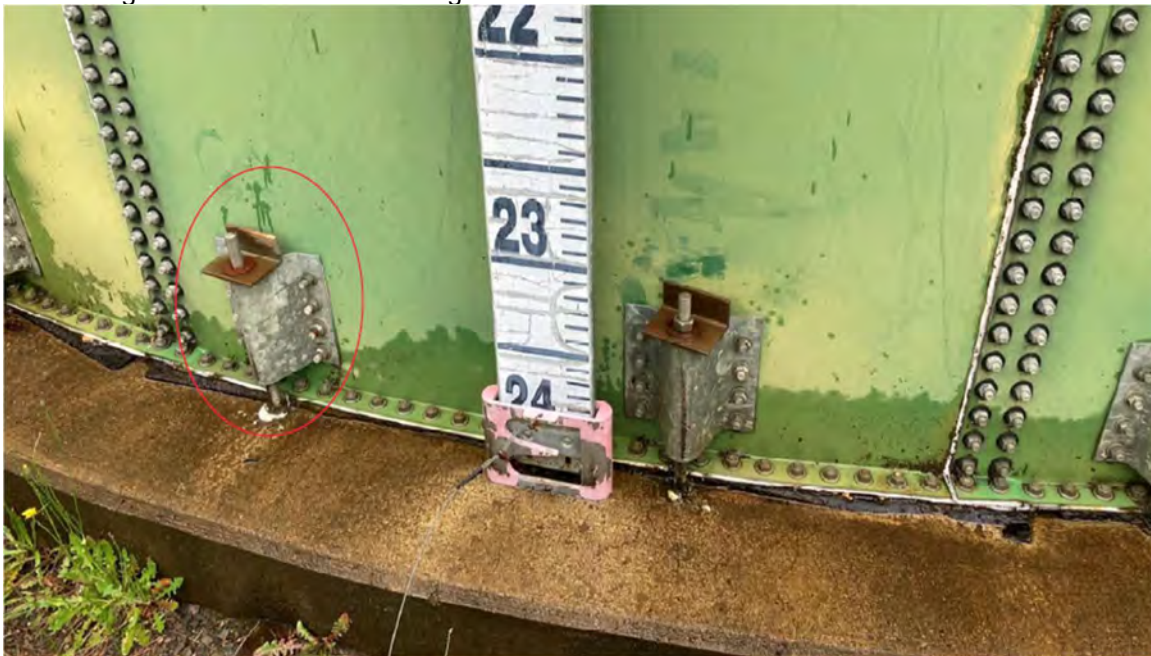
Figure 6.7 Strawberry Reservoir Anchor Bolts
