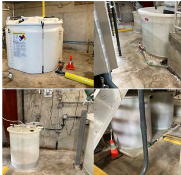
Figure 6.3.4 Tanks without Restraints
