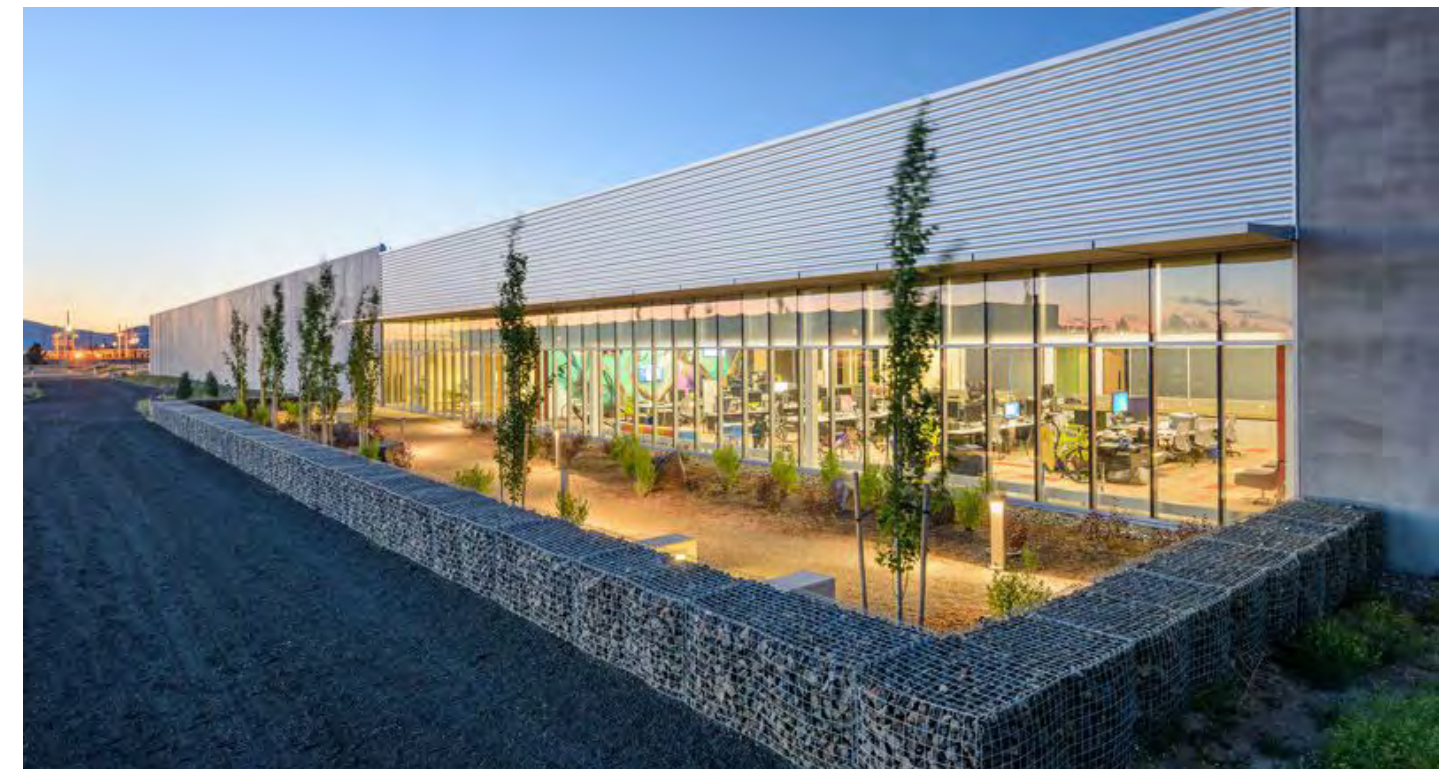
The newest Meta data center in Prineville is LEED Gold certified.
