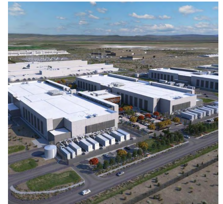
Aerial view of the Meta data center campus in Prineville.
