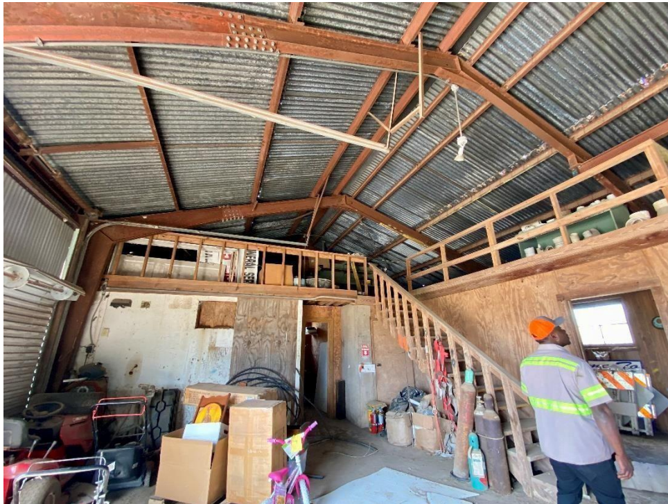
Steel beams inside building
