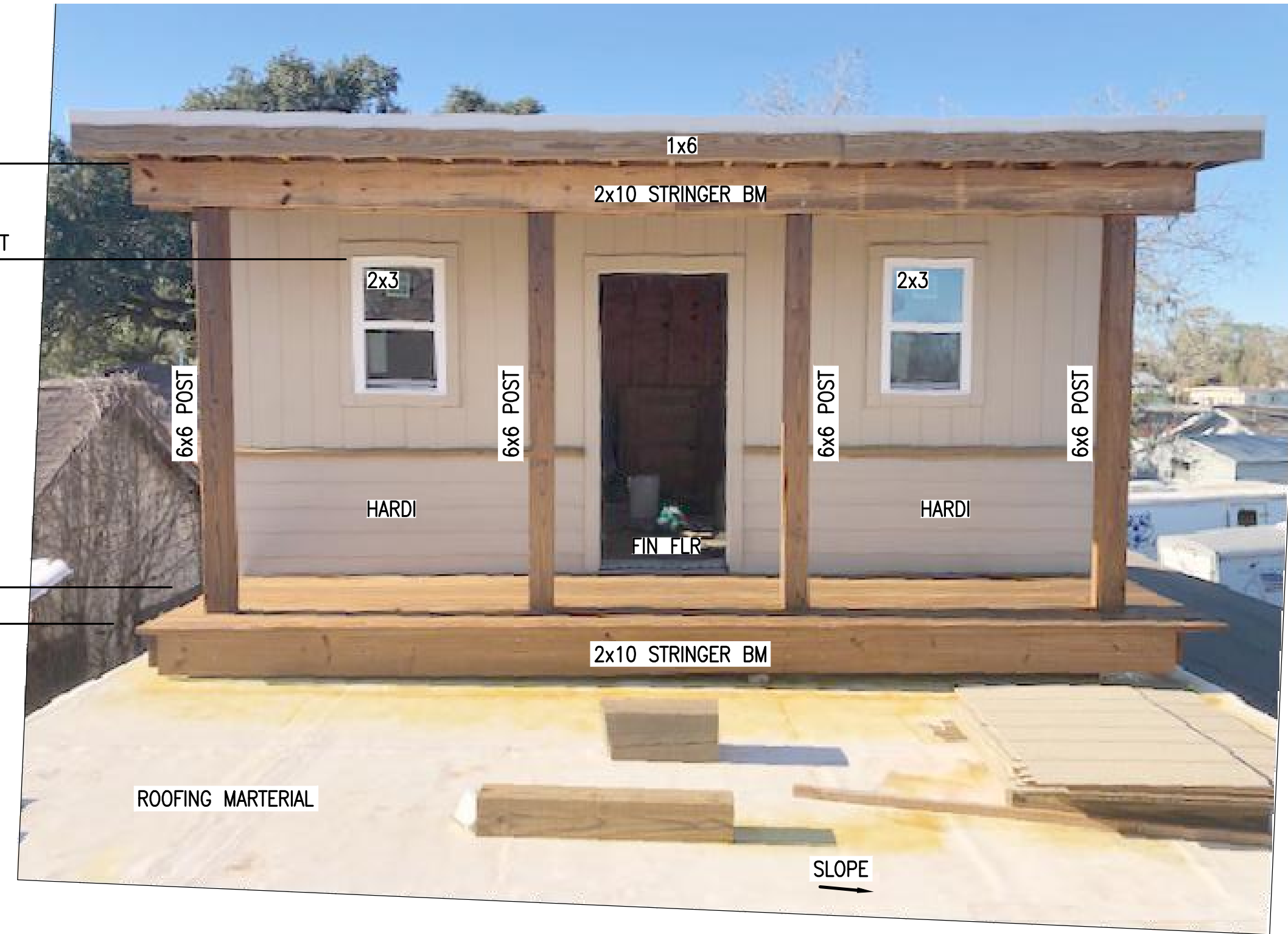
PIC 05 LOOKING NORTH-WEST (SEE DWG J2314-08 & 14)
