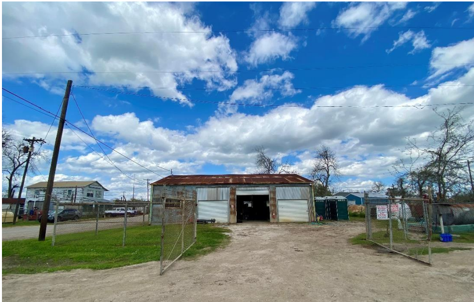
Front of building – additional parking and paving needed.
