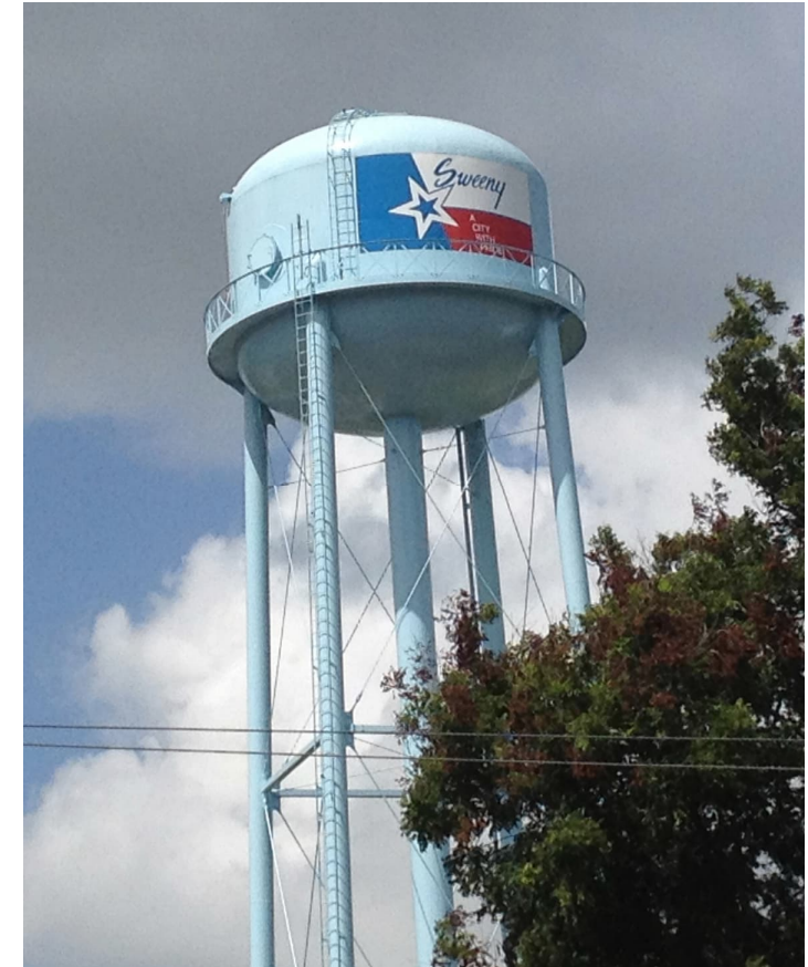
Peach Street elevated storage tank
