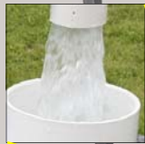
Airgap for backflow prevention
