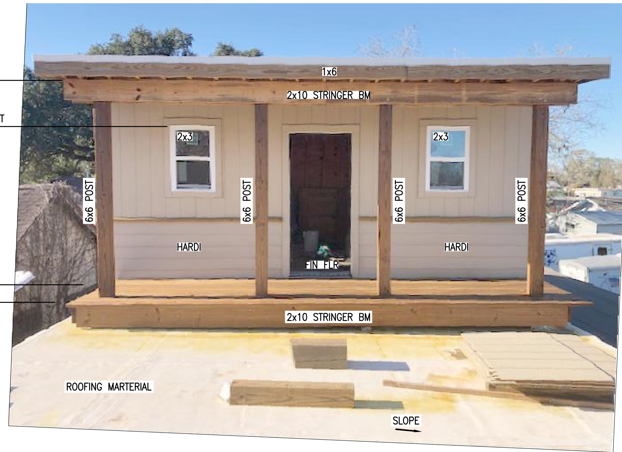
PIC 05 LOOKING NORTH-WEST (SEE DWG J2314-08 & 14)
