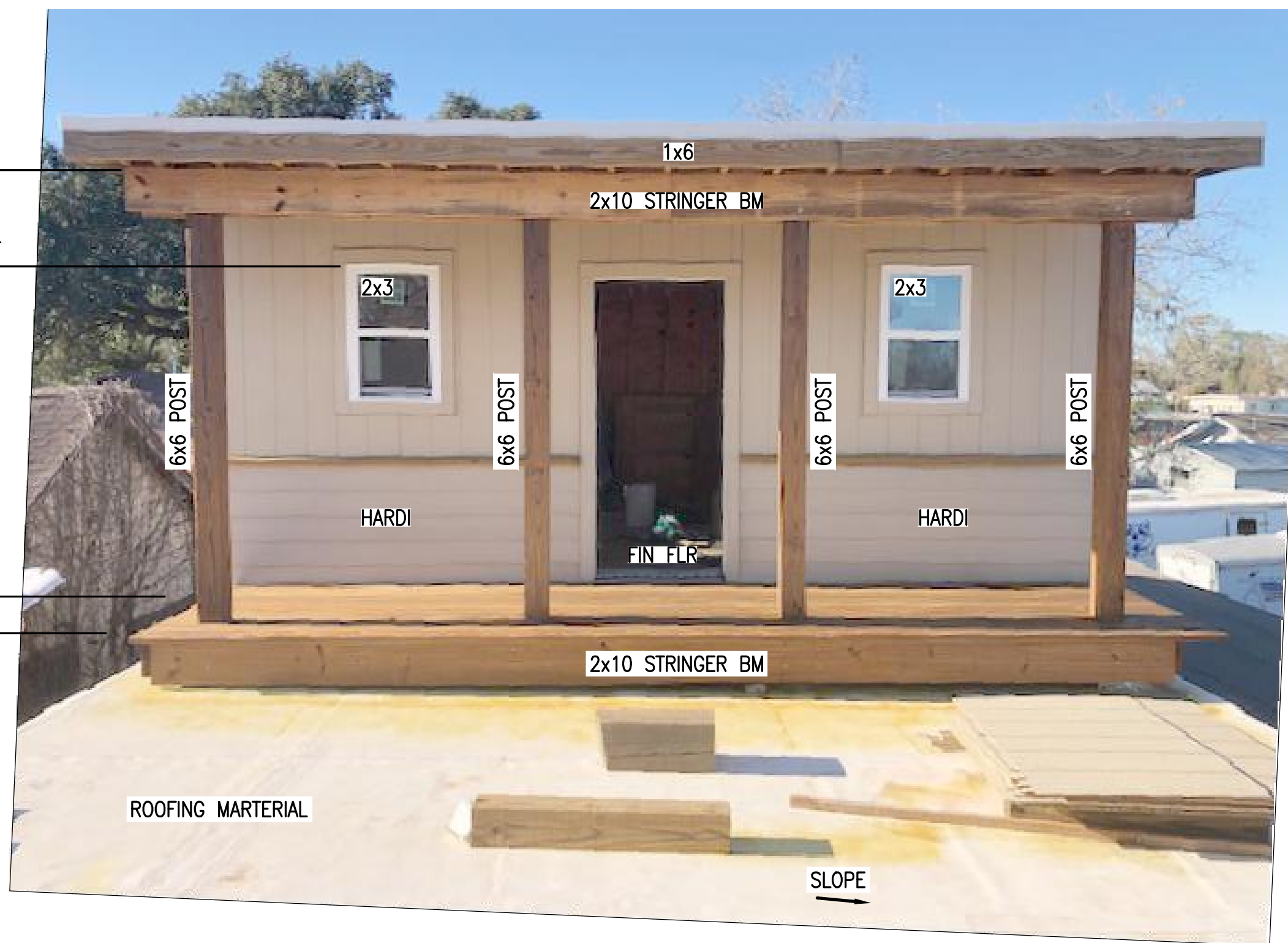
PIC 05 LOOKING NORTH-WEST (SEE DWG J2314-08 & 14)
