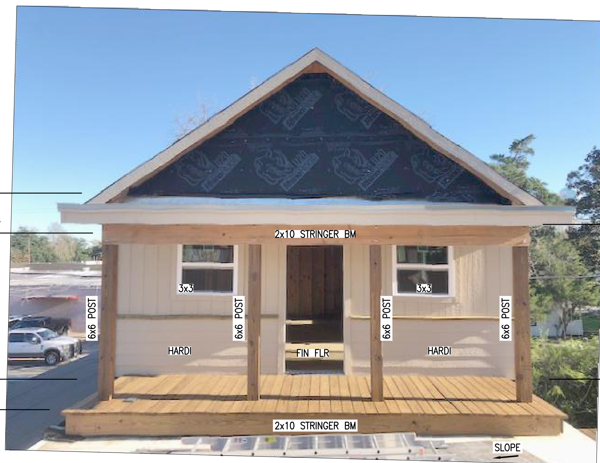
PIC 06 LOOKING SOUTH-EAST (SEE DWG J2314-08 & 14)
