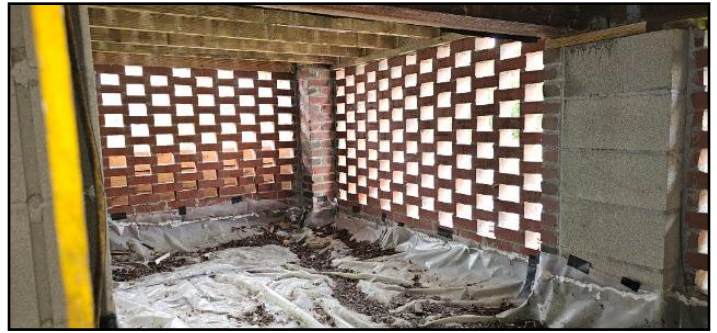
55. Crawlspace below grade
