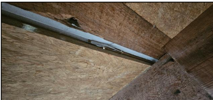
58. Exposed drywall in crawl
