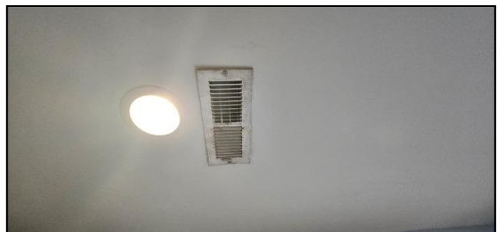
24. Visible growth on register
