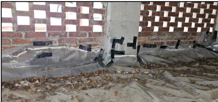
68. Vapor barrier "taped" to wall
