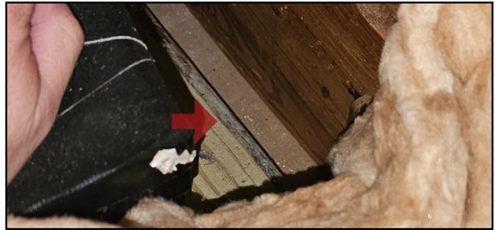
46. Edge of drywall visible from the attic
