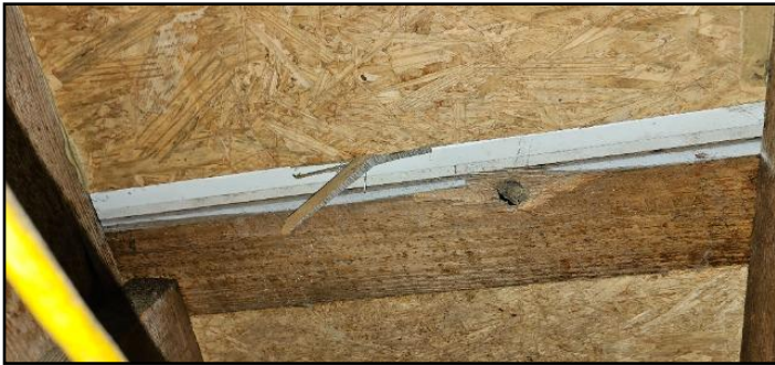
56. Drywall form middle wall visible
