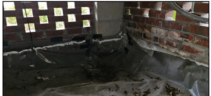
69. Crawlspace below grade
