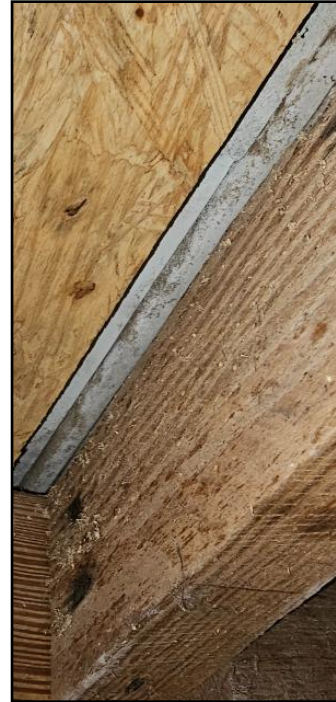
63. Microbial growth on drywall
