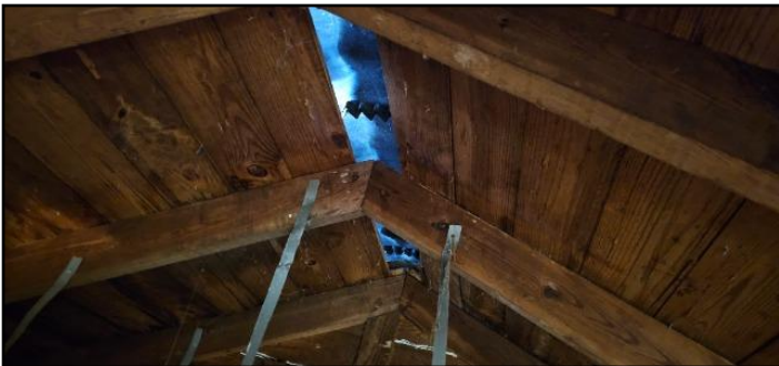
39. Ridge vent looks adequate
