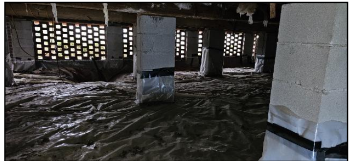
53. Vapor barrier on crawlspace floor
