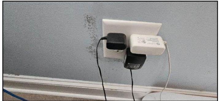
8. Visible growth around outlet
