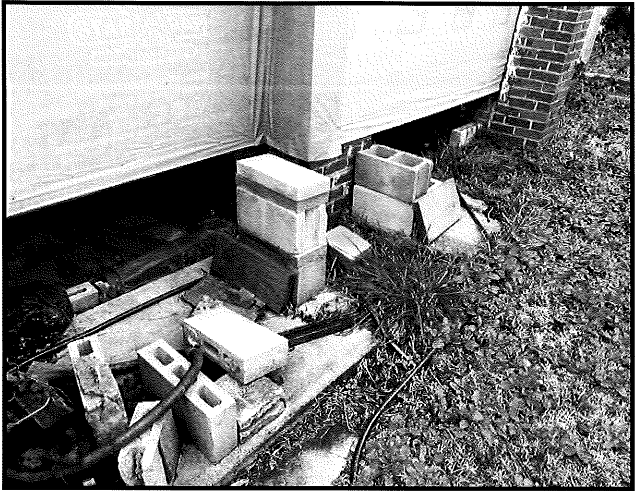
Photo #7: A general loss of masonry infill has occurred along the left side of the home.
