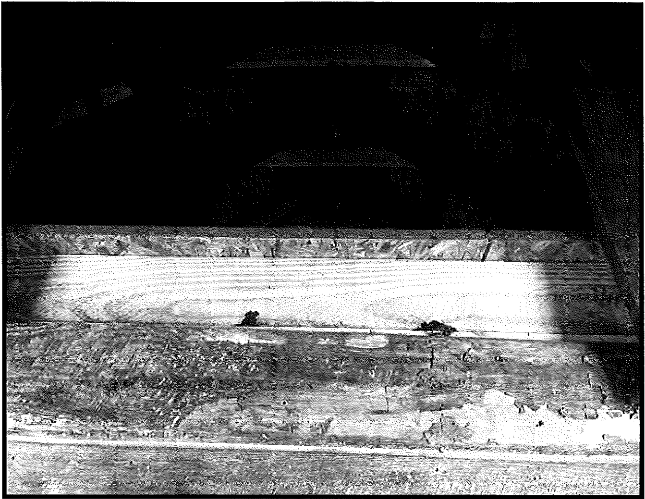
Photo #3: The upper ceiling joists have been reinforced with 2 x 10's and \frac{3}{4} " plywood.
