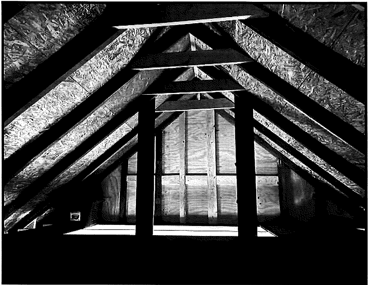
Photo #2: Attic construction: new roof sheathing, gable end wall studs/sheathing, collar-ties, reinforced ceiling joists and 3/4" plywood attic decking.
