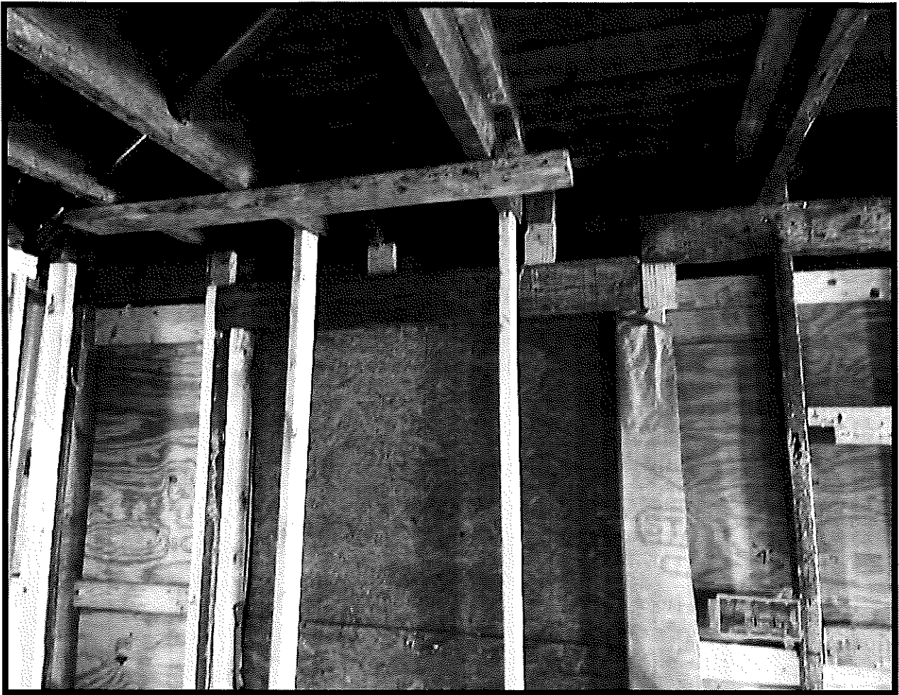
Photo #4: The front door/wall framing support is incomplete.
