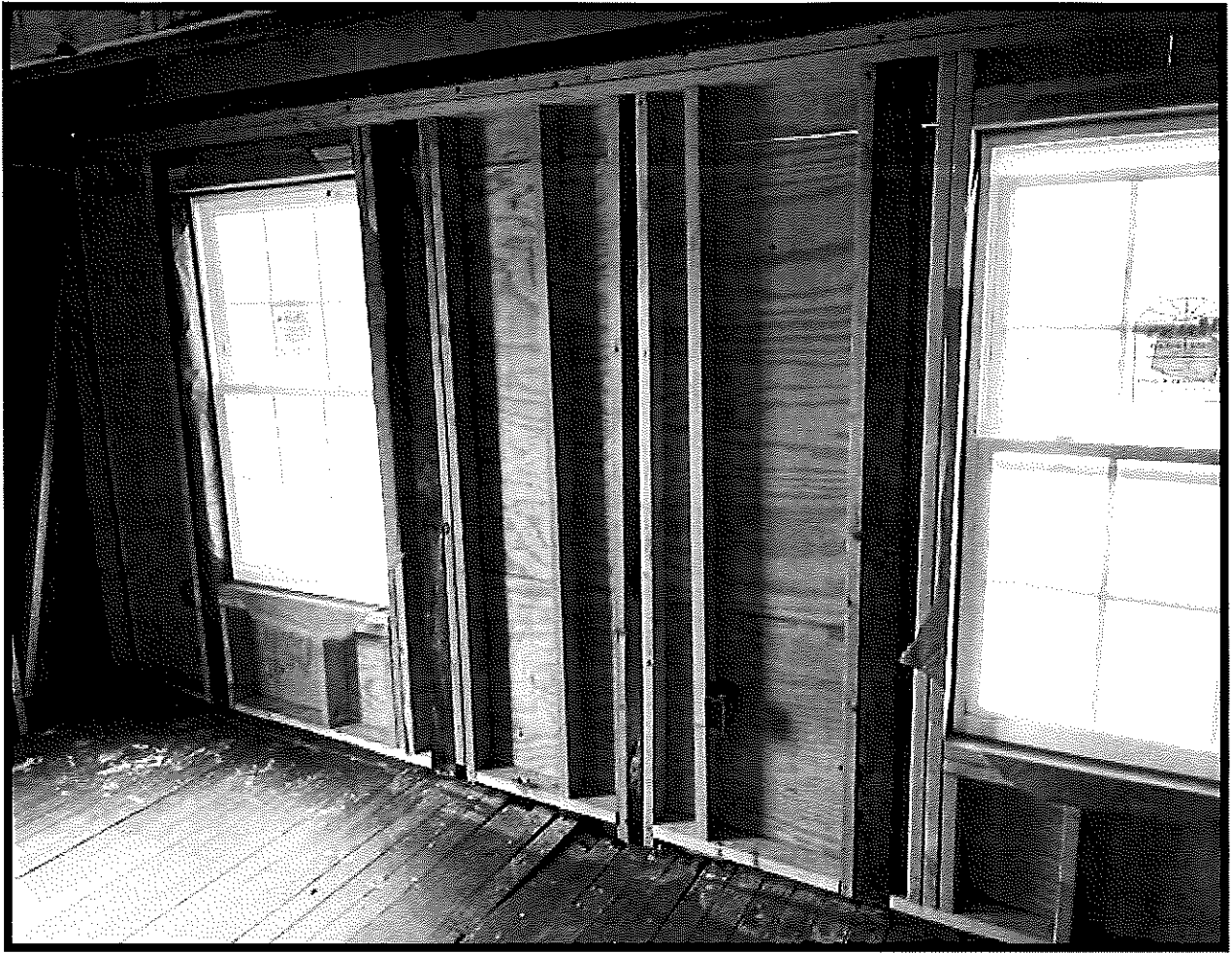
Photo #5: Significantly modified/reinforced stud walls/structural sheathing & new windows.
