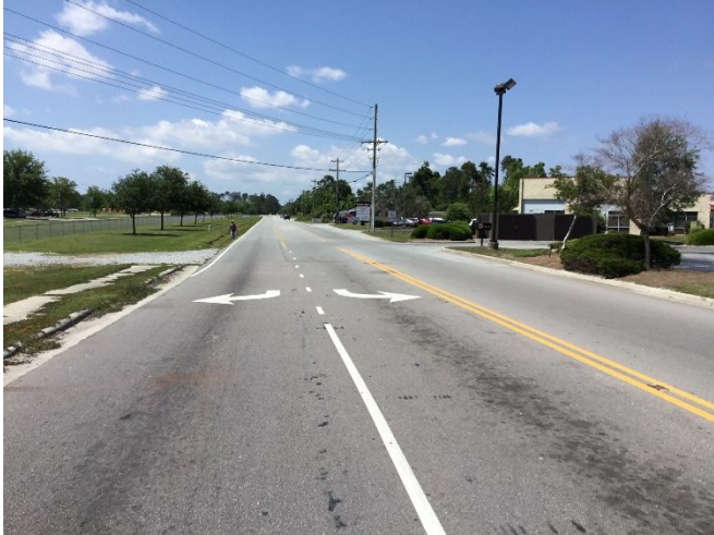
Queens Creek Rd looking south away from NC 24 (Corbett Ave).
