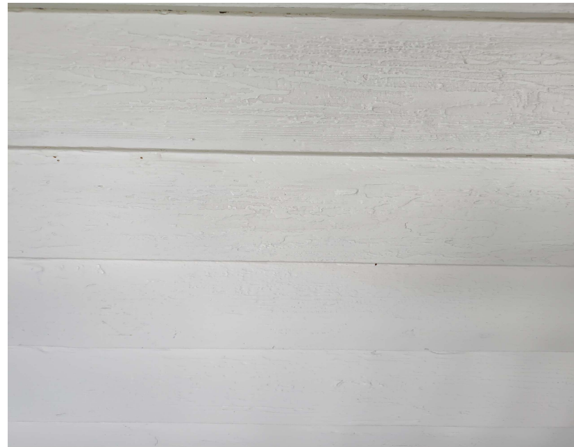
New Fiber Cement Siding for Carport to match Original Siding
