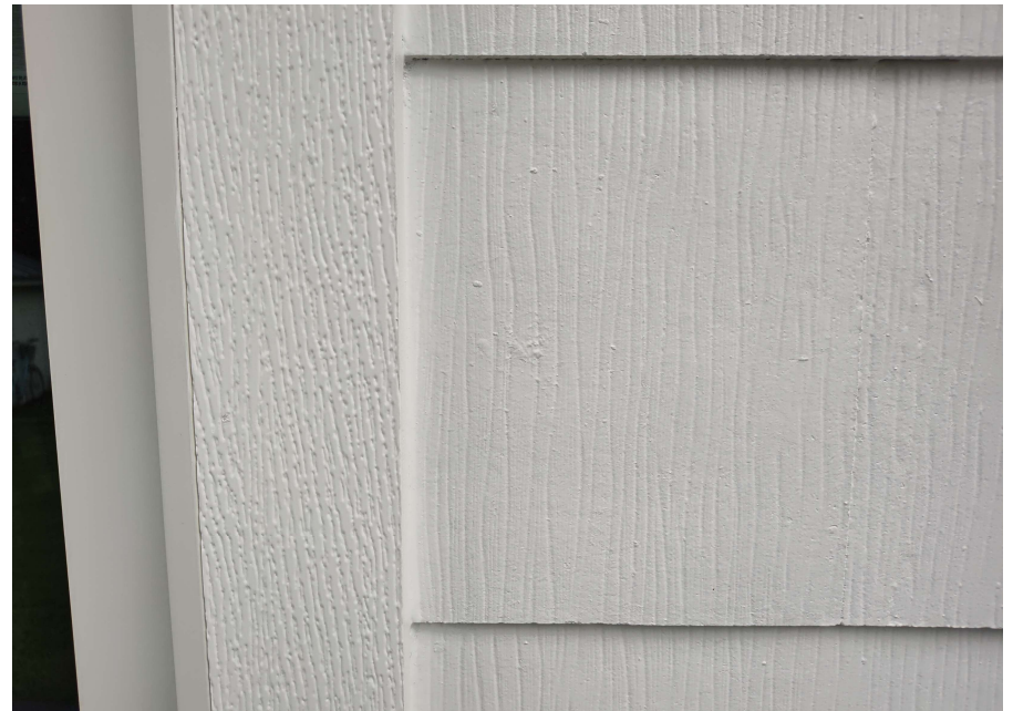
New Siding – Fiber Cement – New Carport
