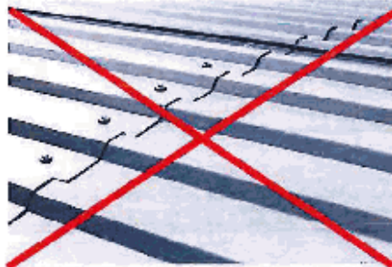
Figure 3.1.5 Inaccurate Metal Roof Example
