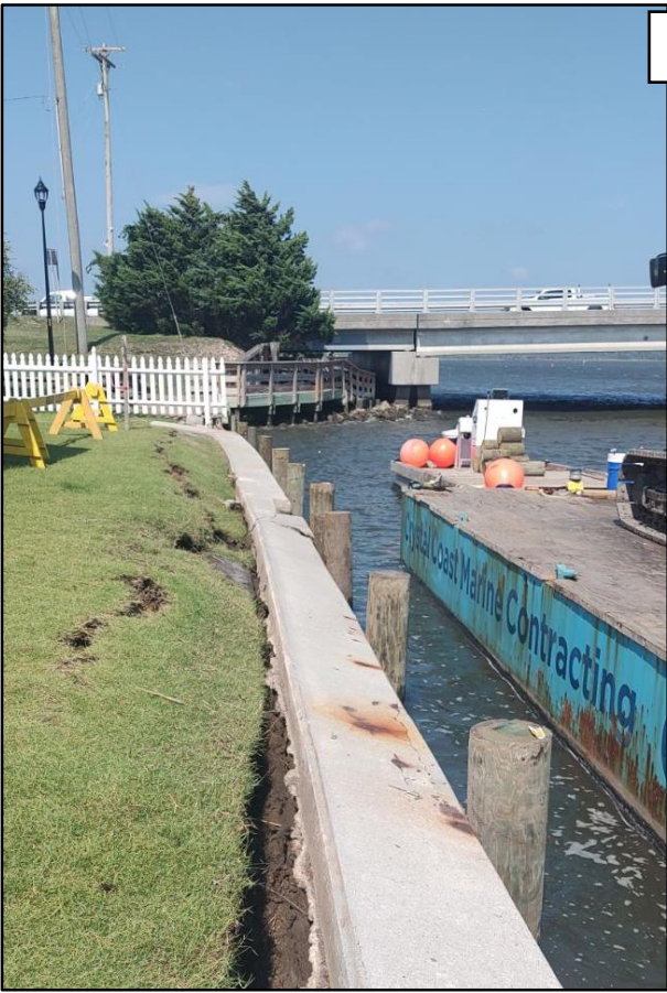
11 pilings added to temporarily hold bulkhead
