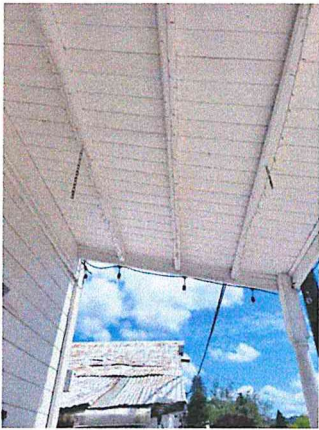
Existing Chains. Sign #2 will be hung from these.
