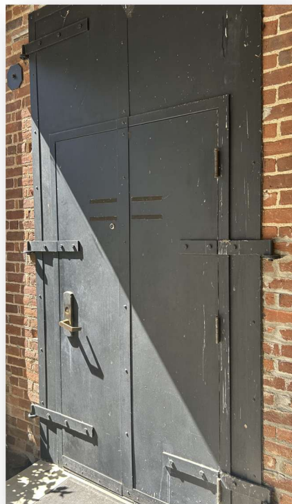
Figure 8 – Front Entry Doors
