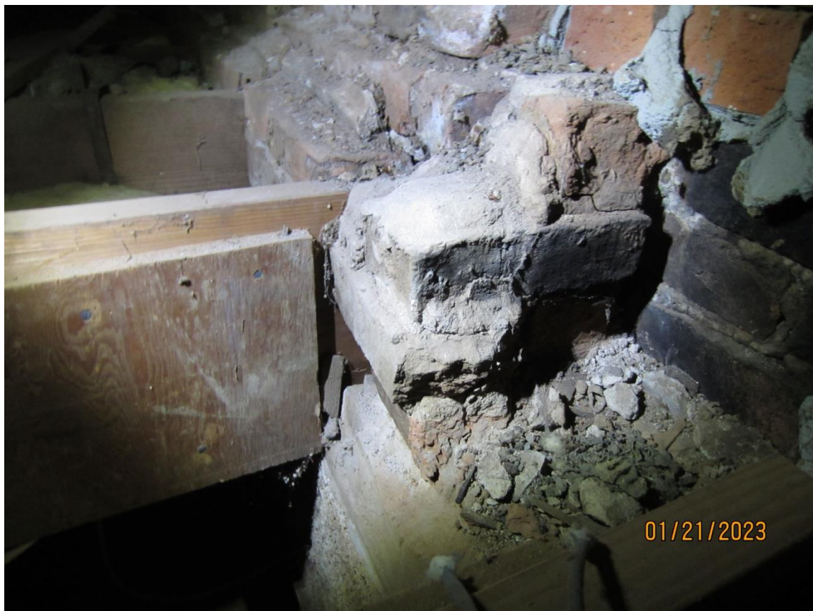
Pic 16 - Loose and missing bricks. Exposed brick head for interior two wythes of wall.
