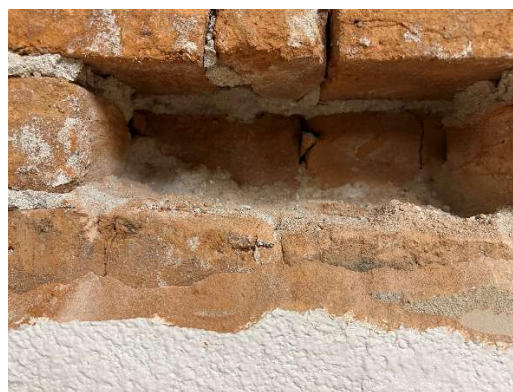
Figure 11 – Mortar and Brick Review – Interior Brick Condition
