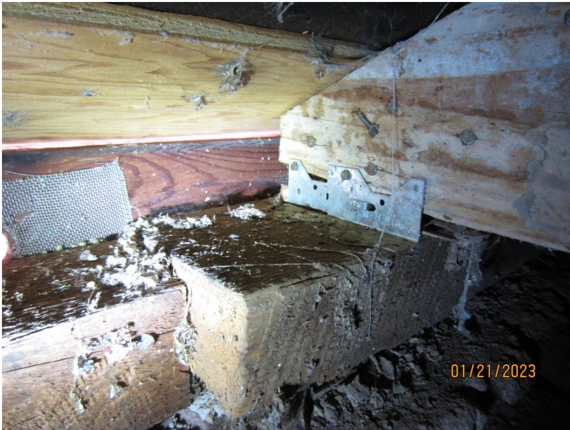
Pic 6 – Roof rafter with low collar tie and Simpson A35 to sill plate at top of wall
