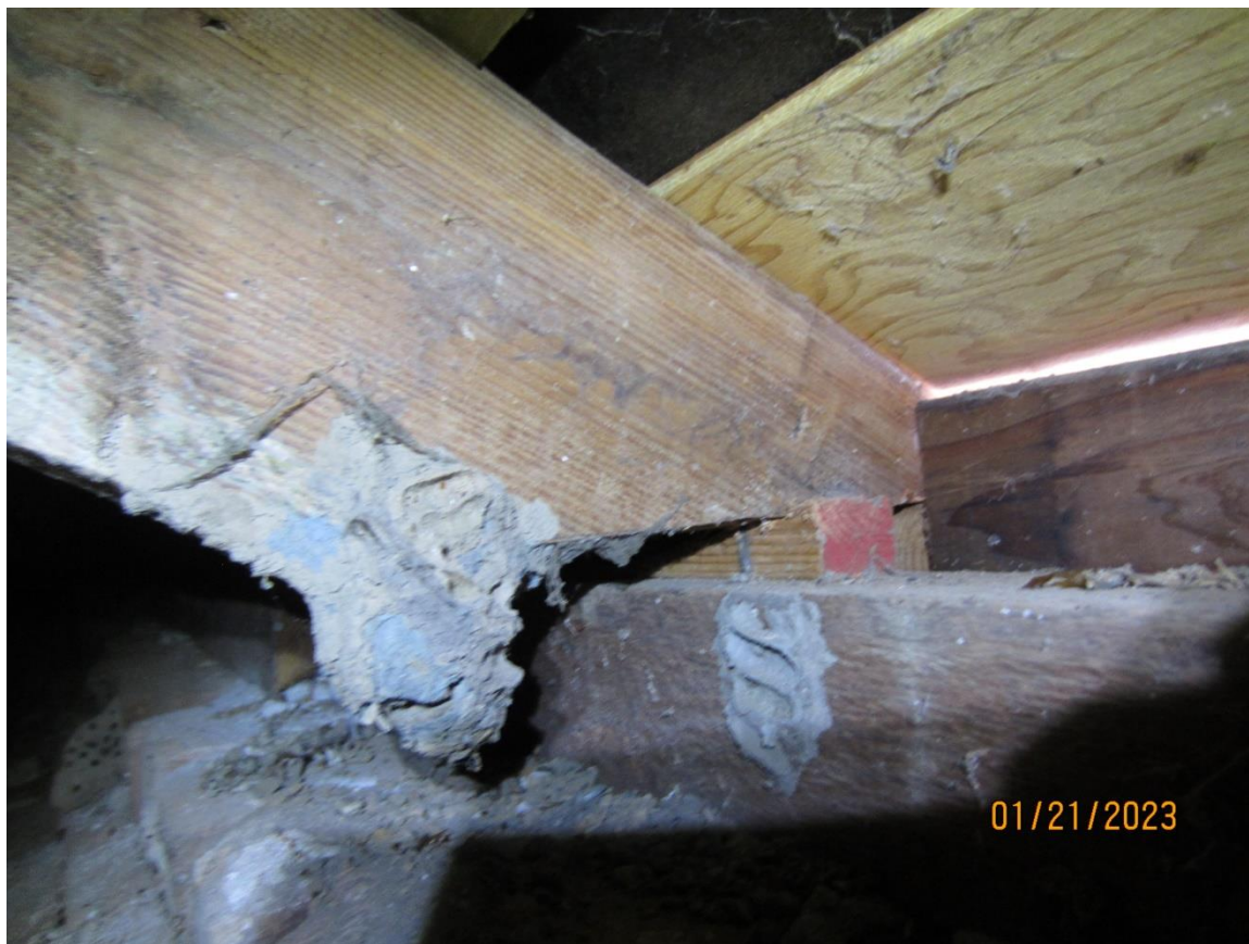
Pic 7 – Roof rafter connection to top of wall at Gridline 2 with spaced sheathing on top
