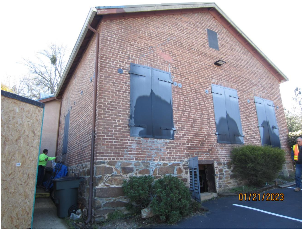
Pic 1- West wall of URM building with access door to crawl space and added anchors each side of existing wall openings.
