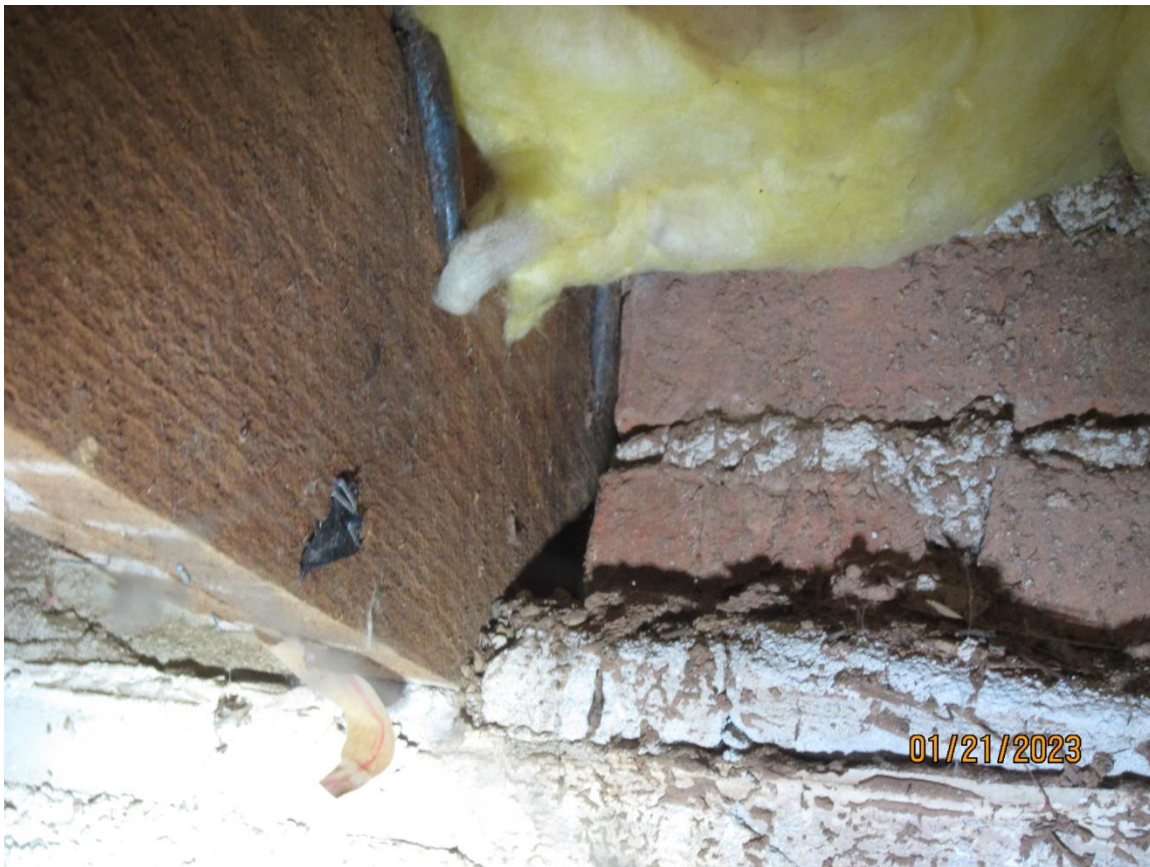
Pic 12 – Dry rot at embedded attic floor joist
