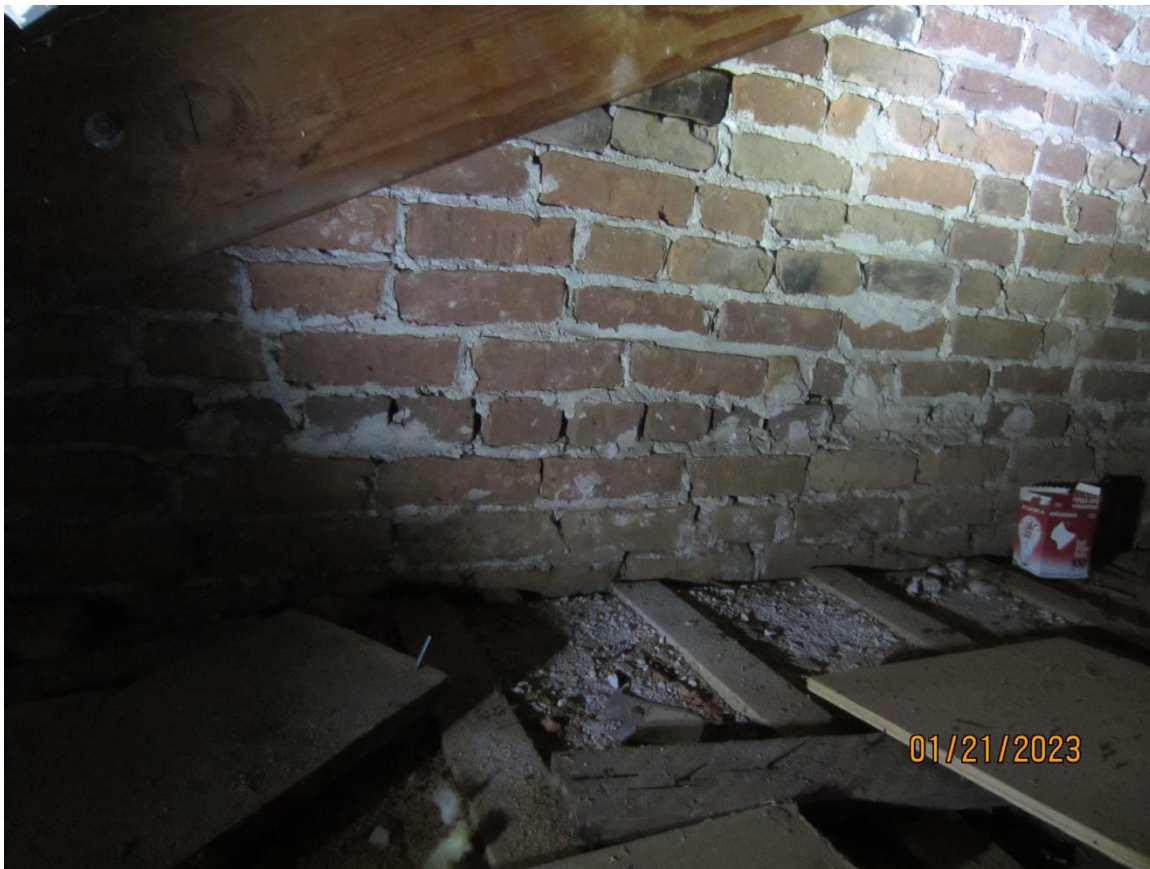
Pic 17 - No wall anchorage at Line B (East Wall) at attic floor level. Attic floor boards removed.
