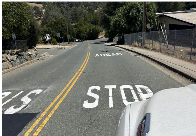
Finished Pavement Markings around Amador High School
