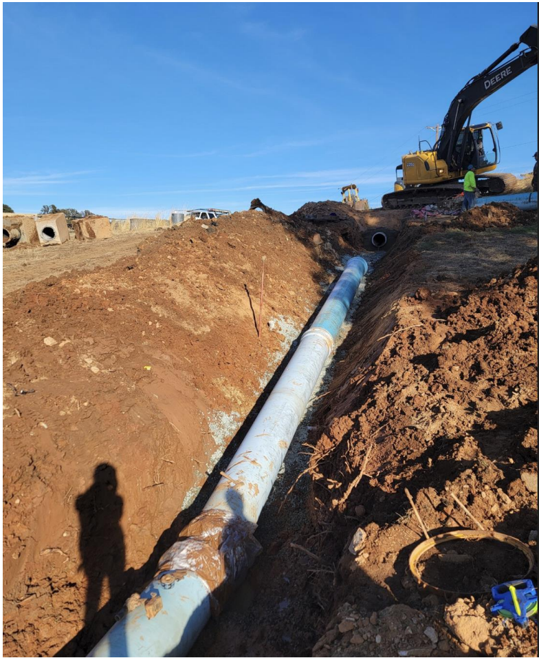
Pipeline repair, full extent
