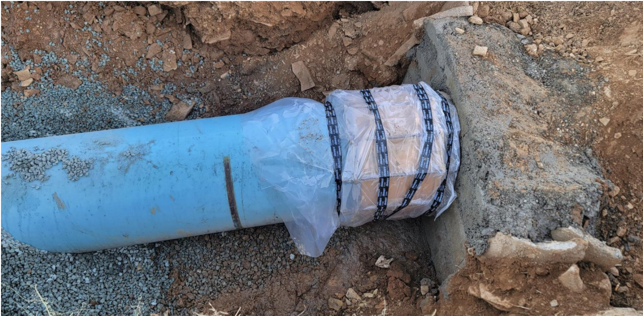
Top Joint repaired
