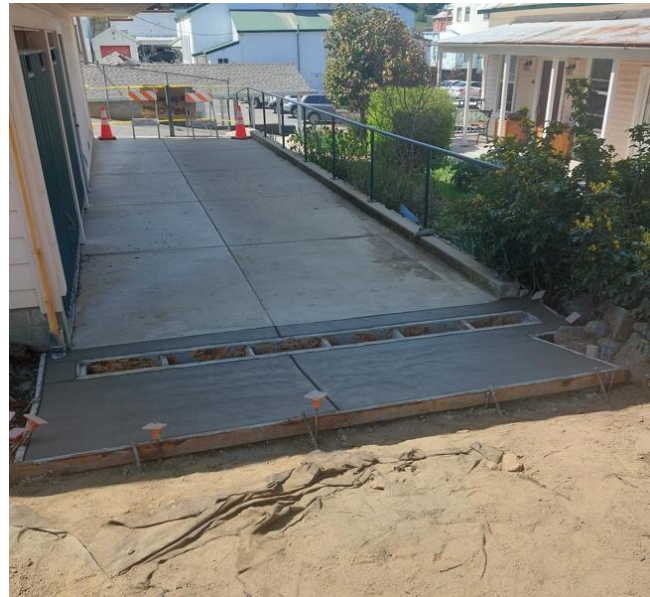
New Curtain Drain
