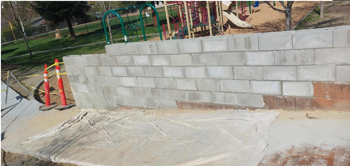
New Wall -not finished (will be covered with stone facade)
