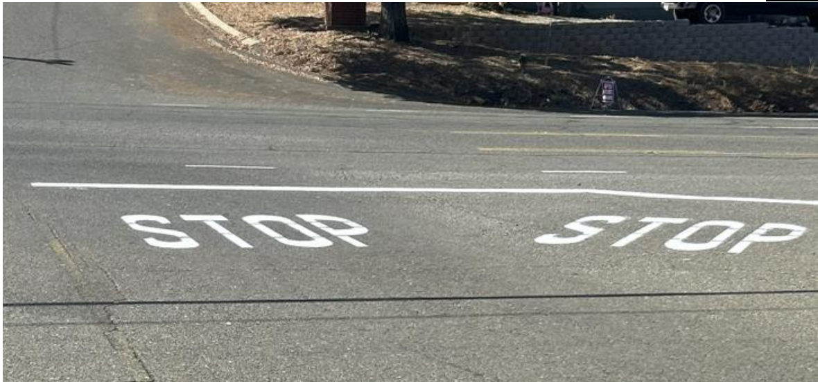
Pavement Marking “STOP” on Lorinda and Old 49
