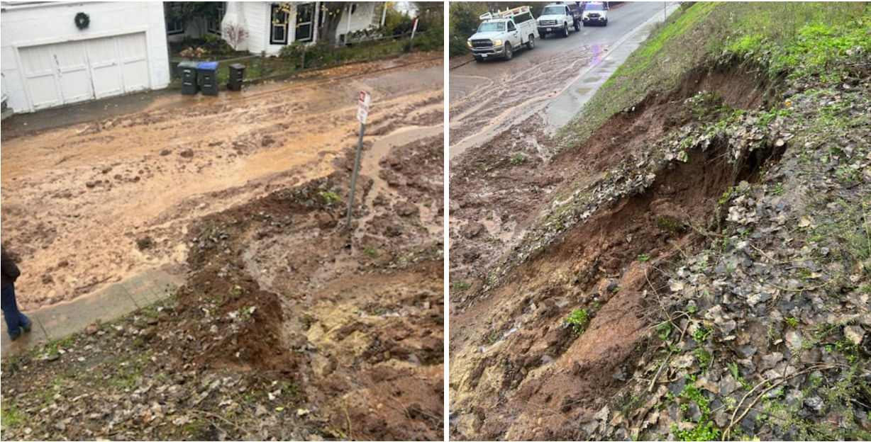
(Hillside collapse due to water leak on school property around 280 Spanish Street)
