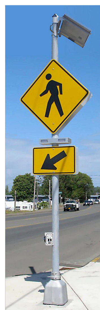
Wrap-around RRFB Light Bar with Required Signage
