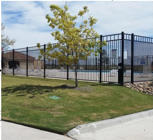
8' HT. ORNAMENTAL FENCE AROUND STADIUM – REPRESENTATIVE PHOTO
